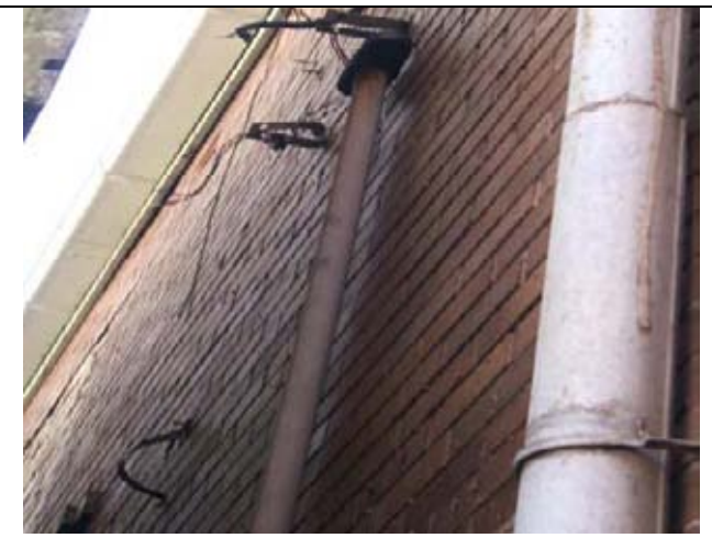
Plate 6: Vent pipe observed on the wall of the RSL site, adjacent to the north boundary of the study area. The pipe is presumably associated with the disused UST in the cellar of the RSL site.
