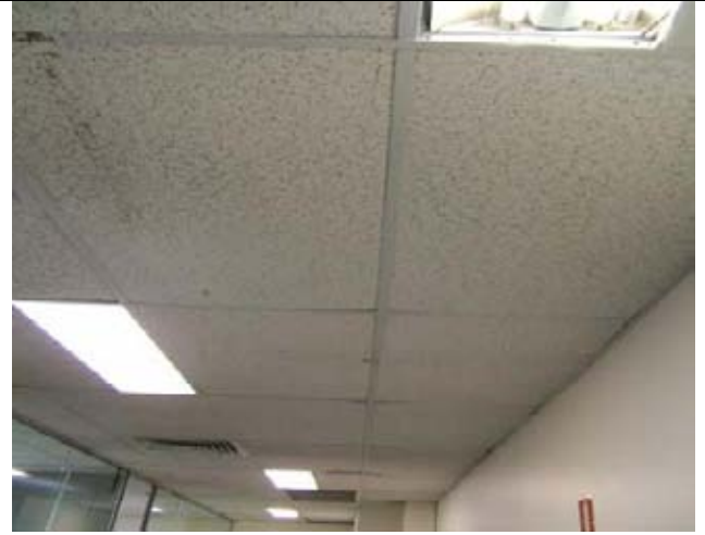
Plate 2: Ceiling panels in the office area at the Travelex site (secured facility).
