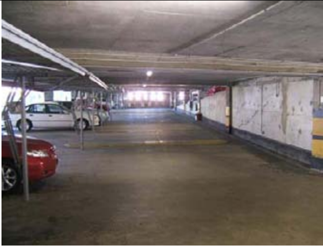
Plate 1: The car park area, above the secured premises.
