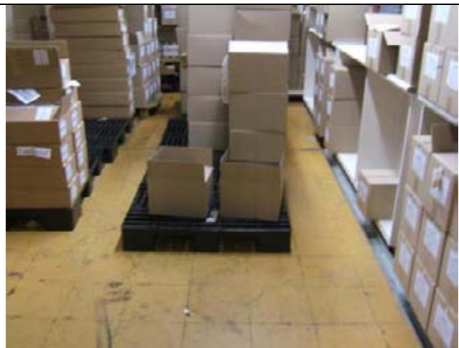
Plate 5: One of Travelex's storage room, paved with brittle vinyl floor tiles.
