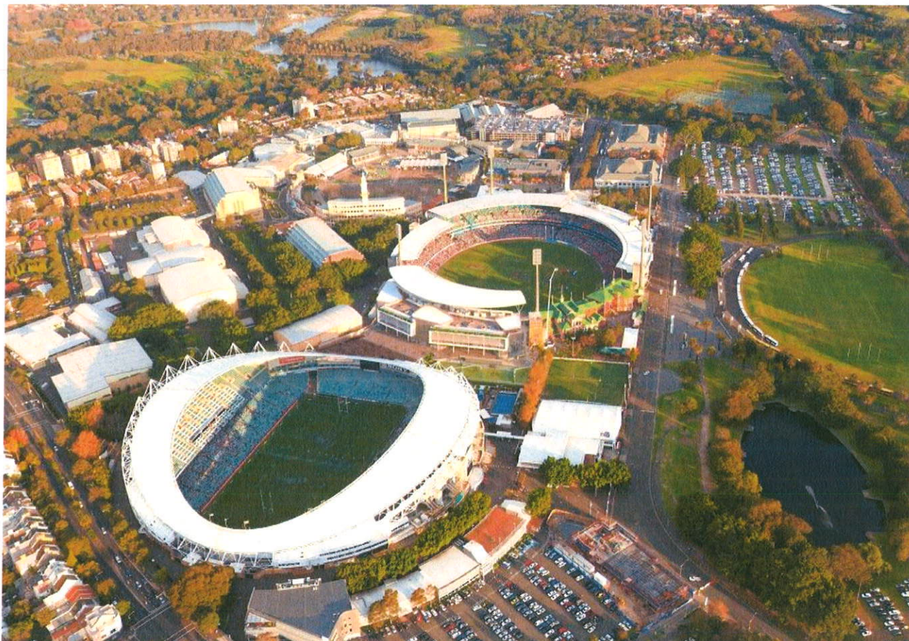
Figure 4 : Photo Montage illustrating relationship between proposed works and Sydney Football Stadium. (Source: EA MP08_0103-Mod2)
