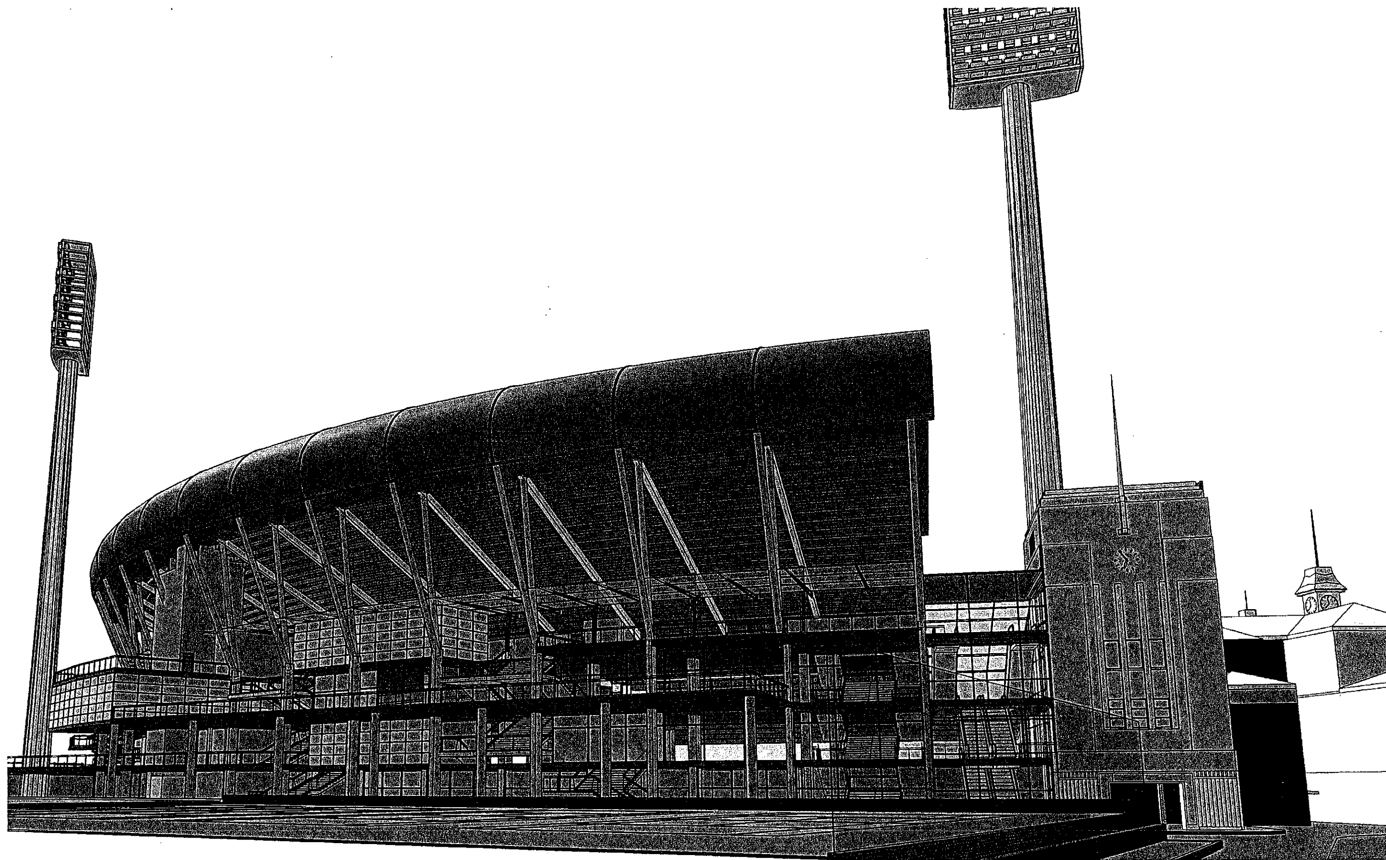
VIEW FROM NORTH SCG STAGE 2 - NOBLE BRADMAN REDEVELOPMENT
