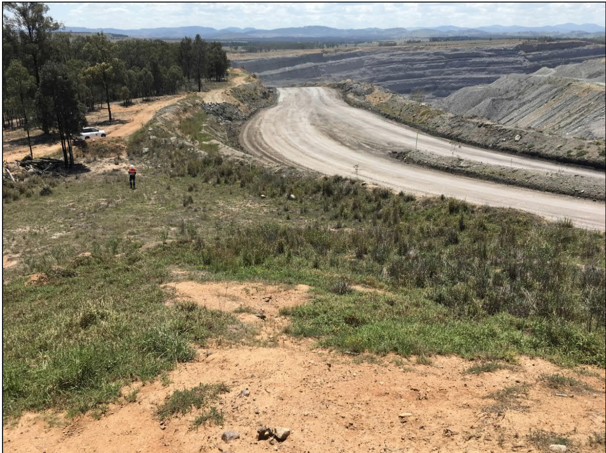
Plate 1 View north from western side of Modification area showing haul road and associated mine activities (Source: AECOM, 2018).
