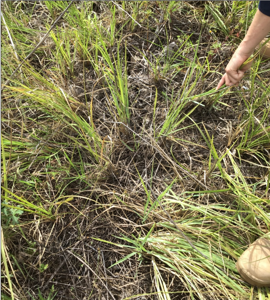
Figure 3: Minor crack observed in fill material of TP2 above Longwall 16.
