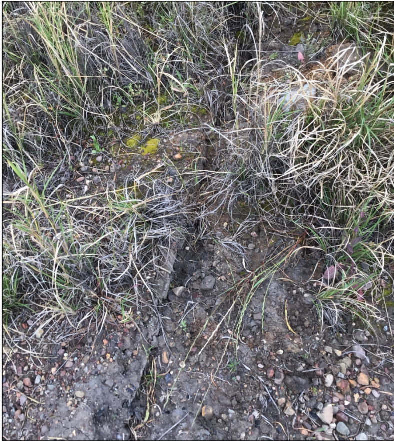
a) Surface crack on 19 October 2020.
