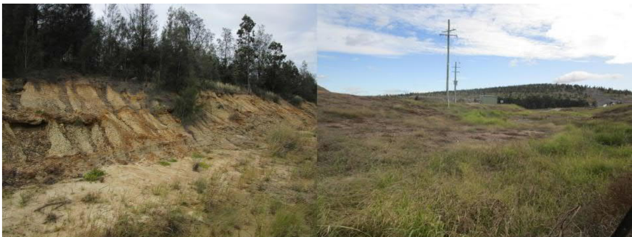
Plate 65 Rill Erosion on Left Bank
