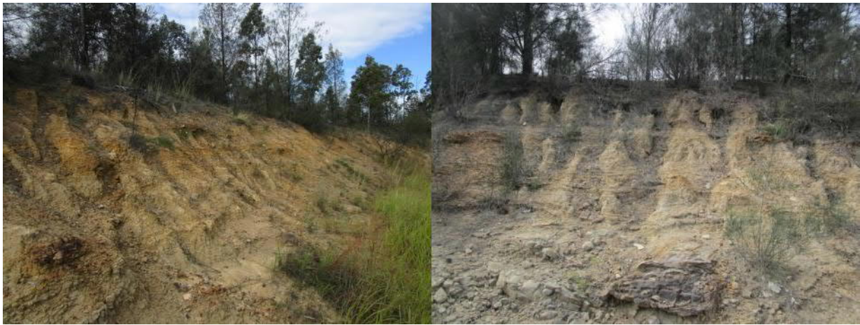
Plate 53 Rill Erosion on Left Bank (1)
