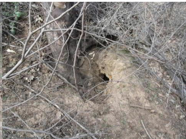
Plate 52 Tunnel Erosion on Left Bank (2)
