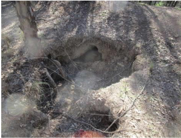
Plate 37 Tunnel Erosion on Left Bank (entry)
