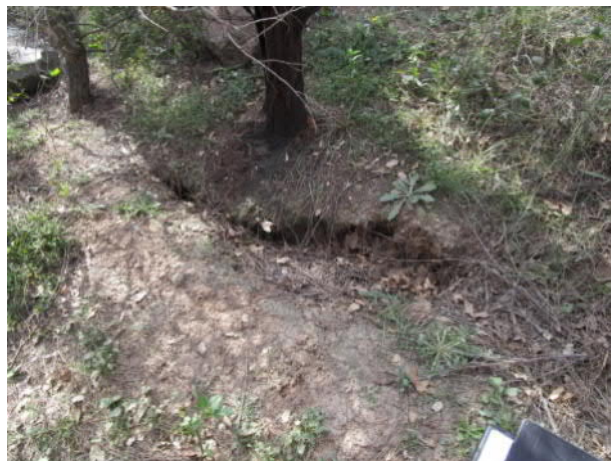
Plate 48 Lateral Crack on Left Bank
