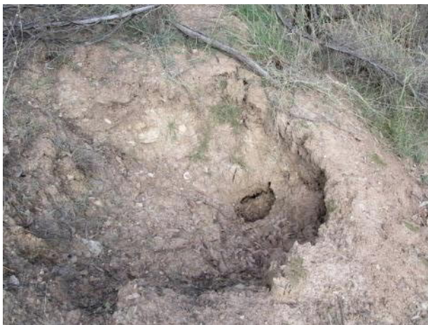
Plate 51 Tunnel Erosion on Left Bank (1)
