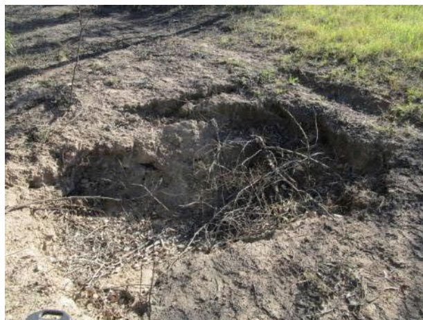
Plate 73 Scour Hole on the Right Bank
