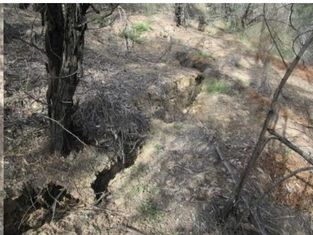
Plate 50 Lateral Crack on Left Bank (2)
