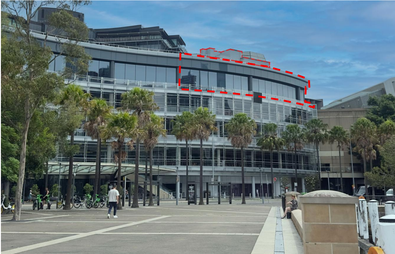
Figure 2 The site as viewed from Pirrama Road (site location outlined red)
