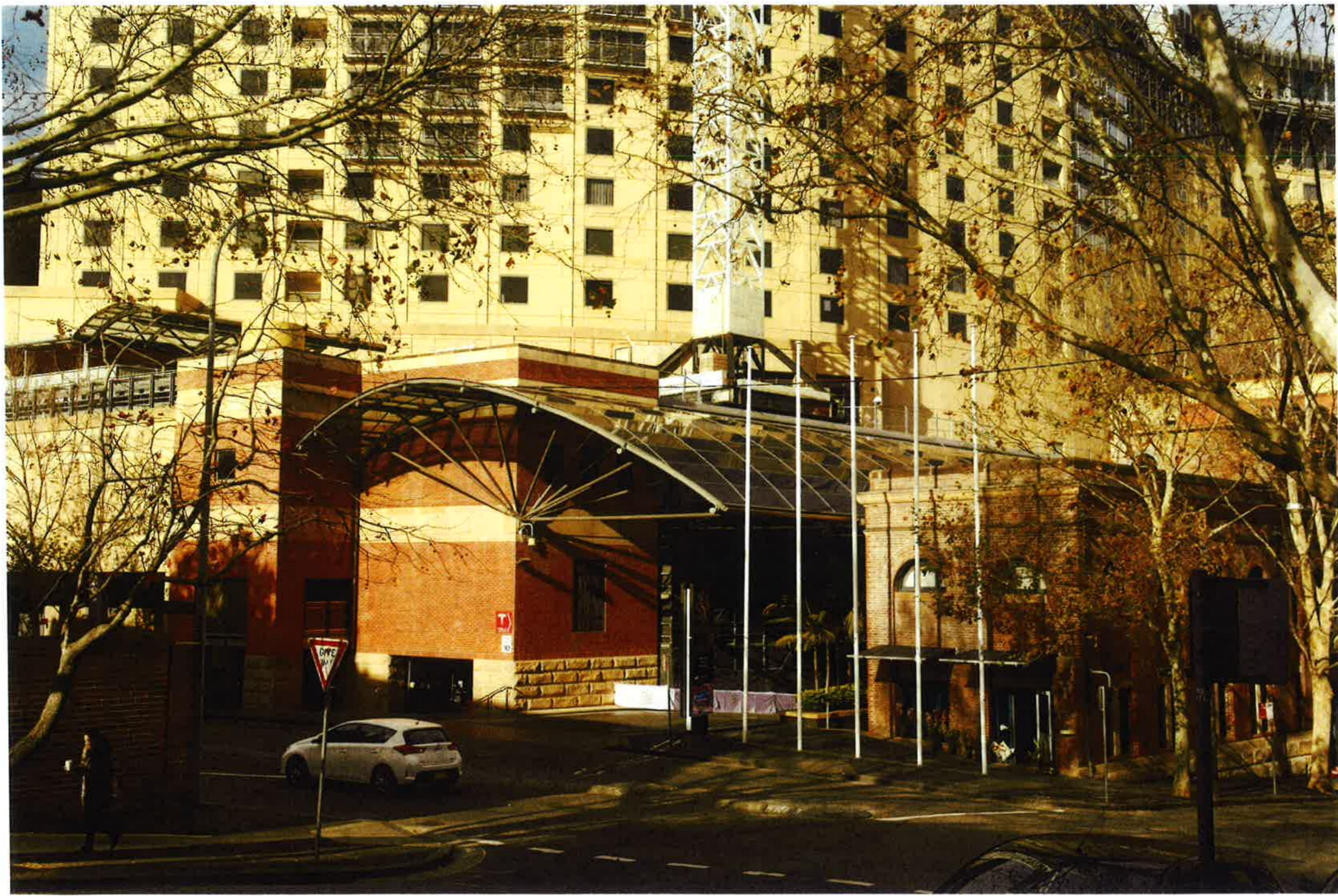
1 EXISTING NORTH WEST VIEW 1:200
