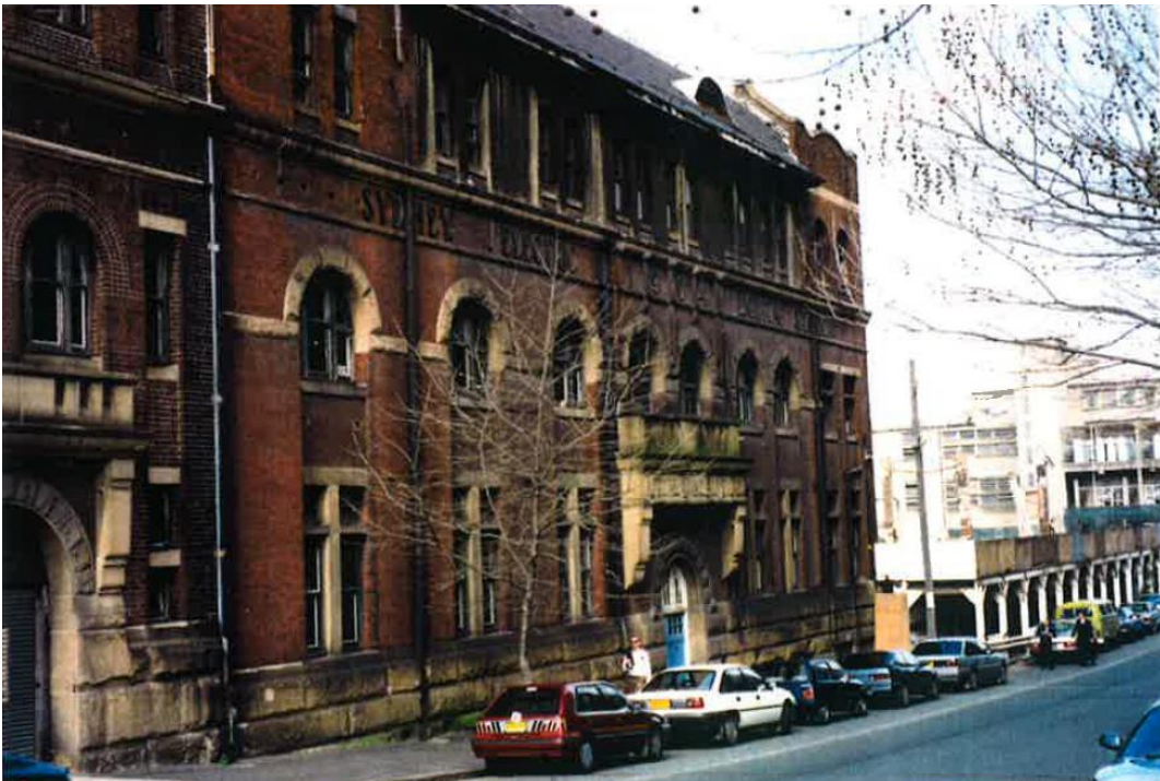
Picture 108 – West elevation to Pymont Street Source: Conservation Management Plan (Tanner) 1994
