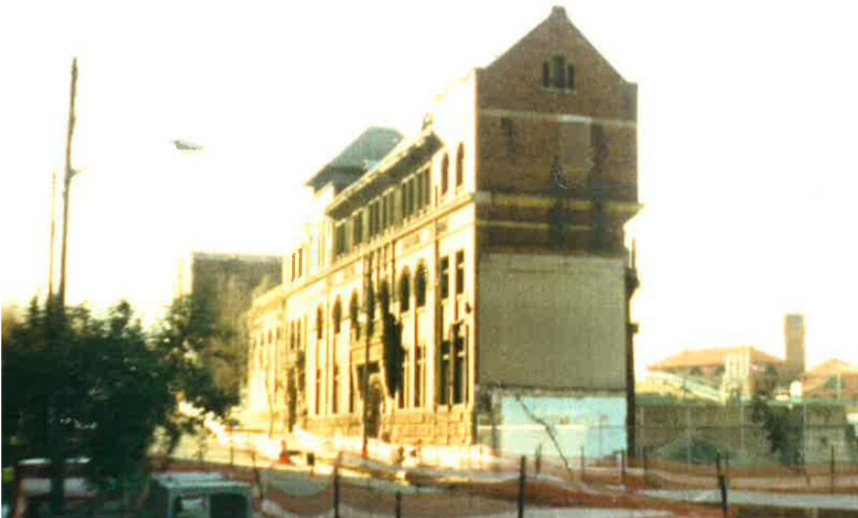
Picture 110 – South elevation of the Offices of the Sydney Electric Lighting Station Source: Conservation Management Plan (Tanner) 1994
