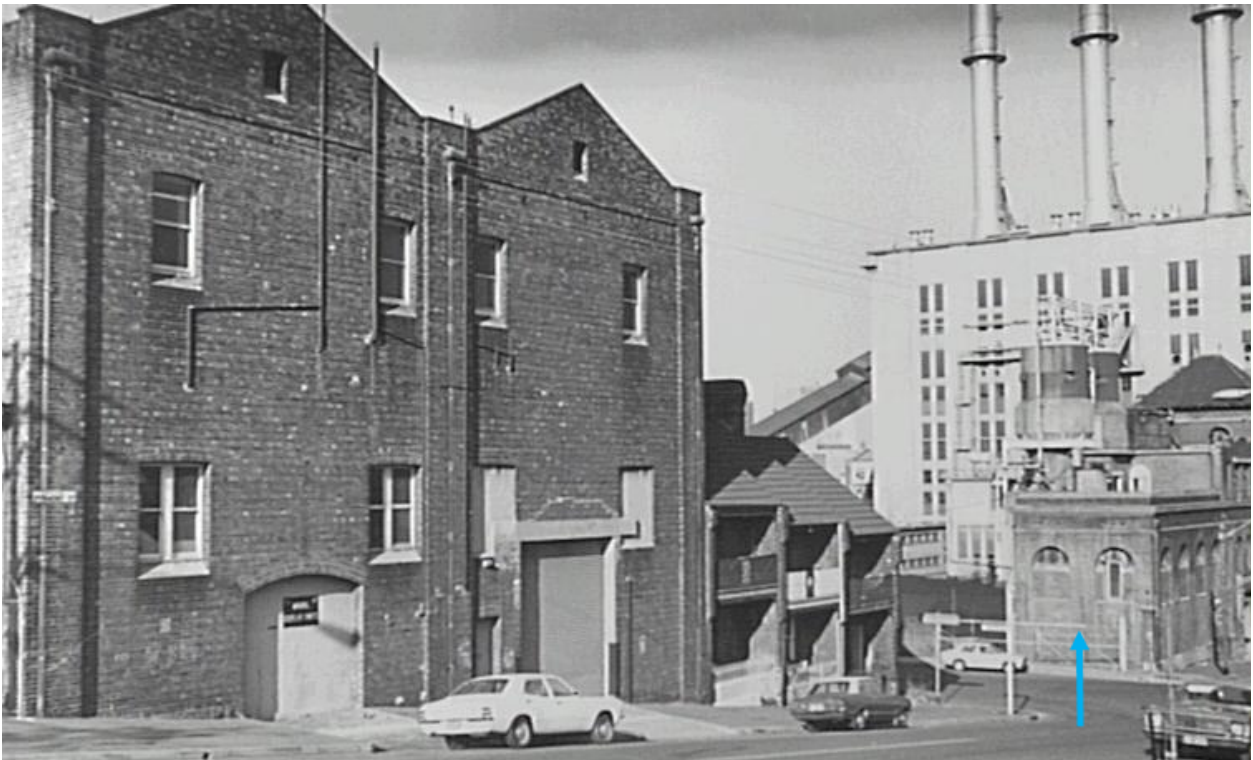
Figure 54 – C1970. Looking south east down Pymont Street from cnr of John Street. The Boilerhouse to the east of The SELS (blue arrow) had been removed by this time.
