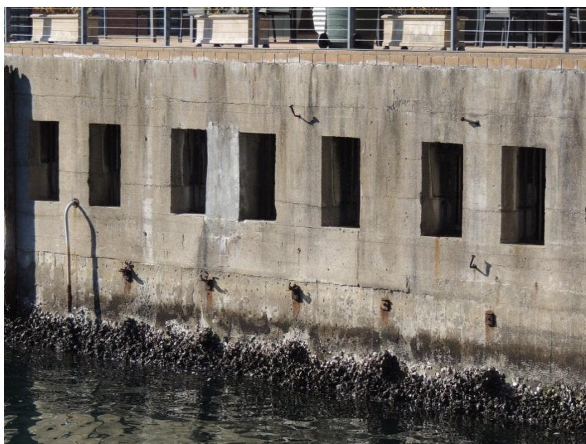
Figure 5.3 Location of existing seawater inlet culverts at the head of Jones Bay
