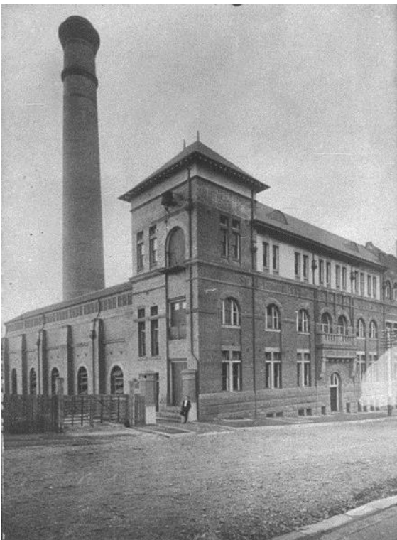
Figure 12 – c1905. Northern extent of the original 1904 section of the Sydney Electric Lighting Station” Powerhouse – Pyrmont
