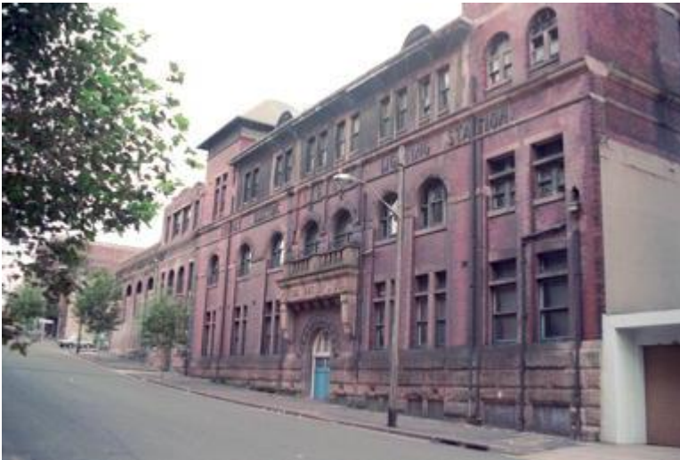
Figure 21 - c1990s. Western façade of the Pyrmont Power Station.
