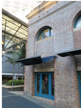
Picture 3 – Part of the northern façade of the SELS Building.
