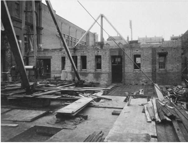
Picture 8 – 1921. View west towards the eastern façade of The SELS under construction.
