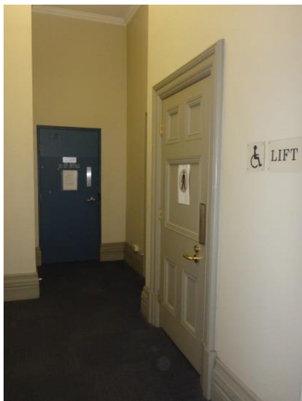
Picture 16 – View towards the fire door on the southern wall of The SELS. The door to the right to the Men's bathroom constitutes later fabric.
