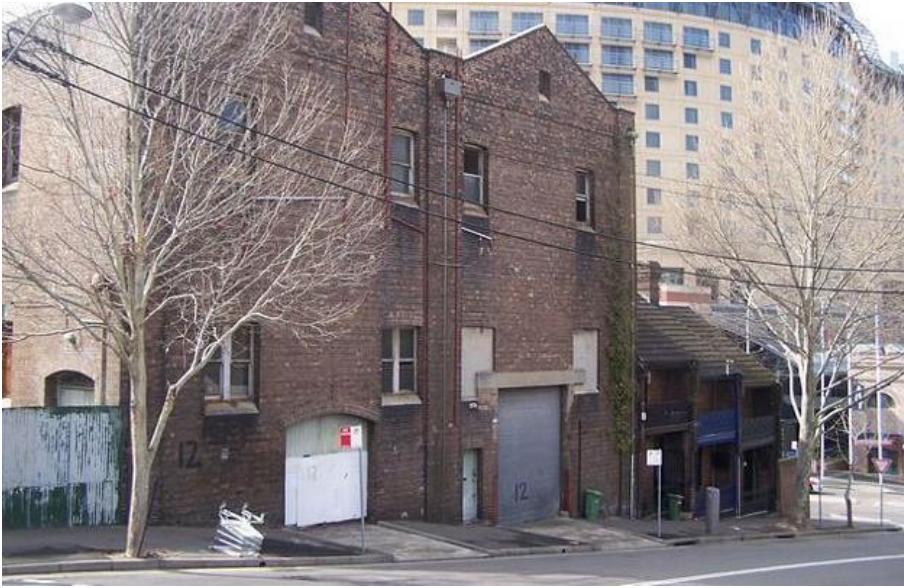
Figure 8 - Western elevation of the “Slades Building” and adjacent terraces.
