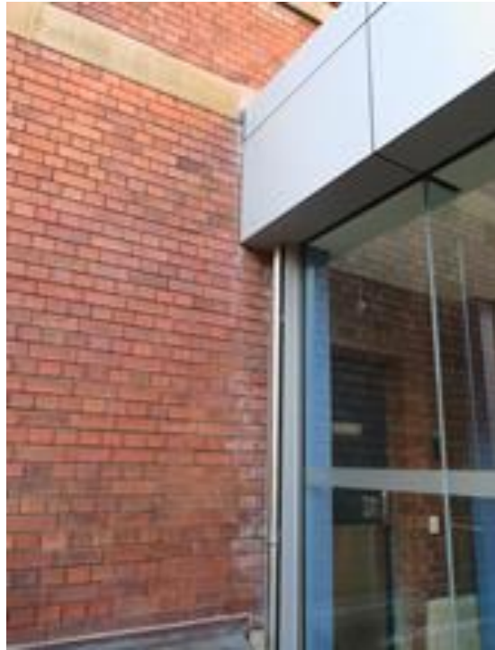
Picture 13 – View of the junction between The SELS and the contemporary structure adjacent which has externalised part of the southern façade of The SELS.
