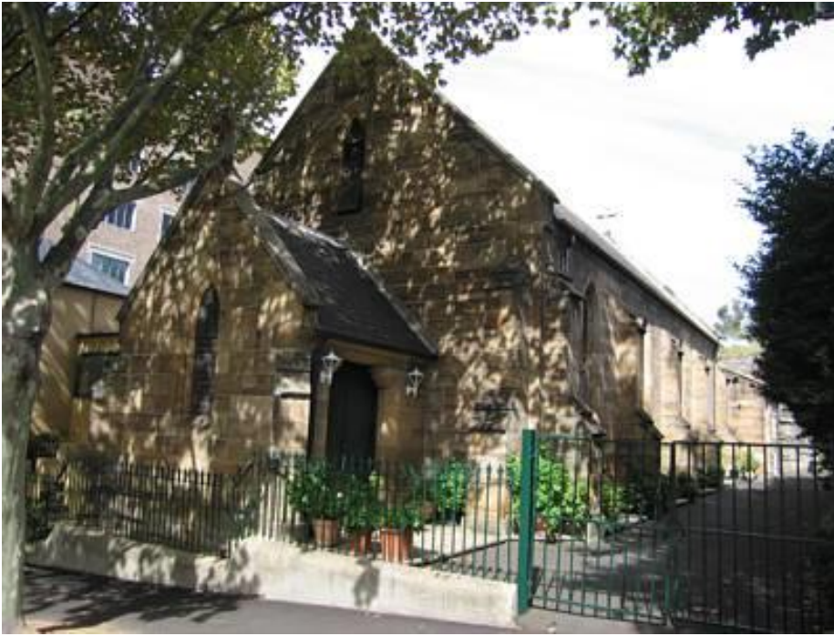
Figure 9 - Eastern elevation of St Bede's School Church
