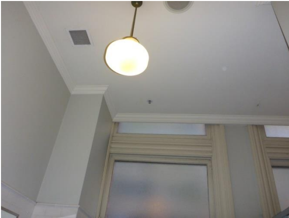
Picture 18 – Suspended ceiling in the women's bathroom.
