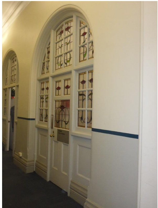
Picture 24 – View south down corridor towards office doors.
