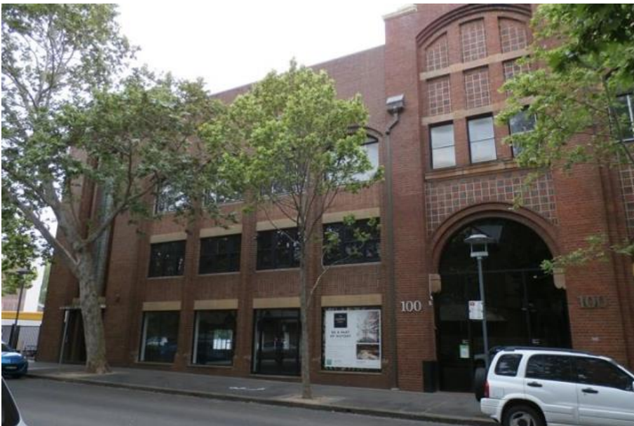
Figure 7 - Western elevation of the former woolstore “Shute, Bell, Badgery and Lumby”.
