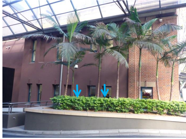
Picture 9 – Current view towards the eastern façade of the SELS. Later openings are identified by arrows.
