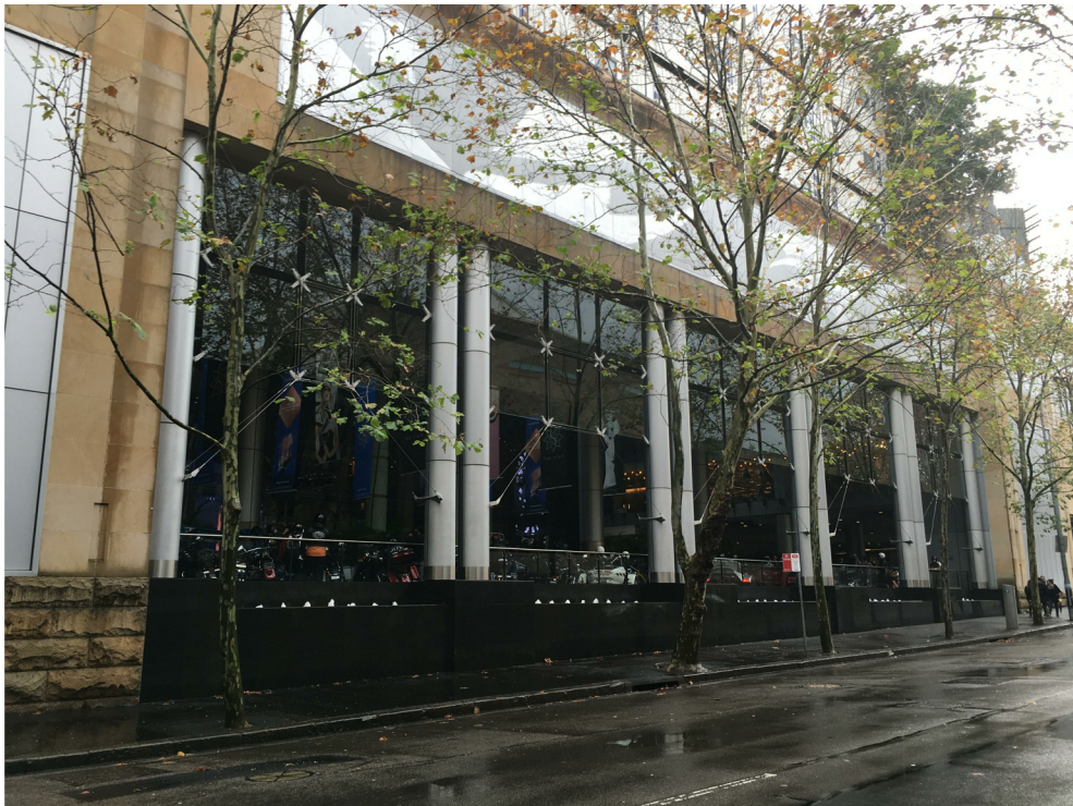
CURRENT VIEW FROM PYRMONT STREET
