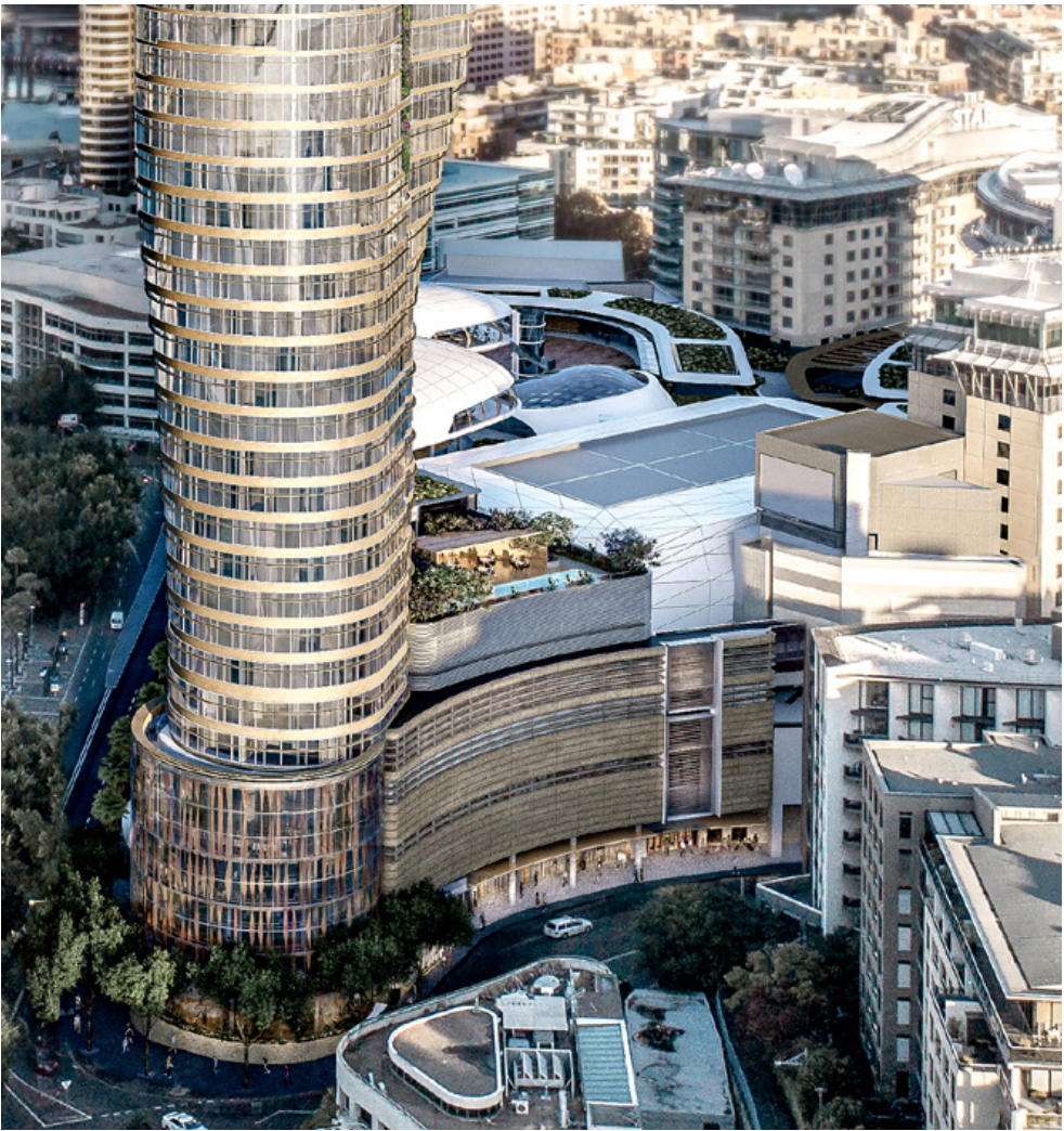
Sandstone Facade along Jones Bay Road
