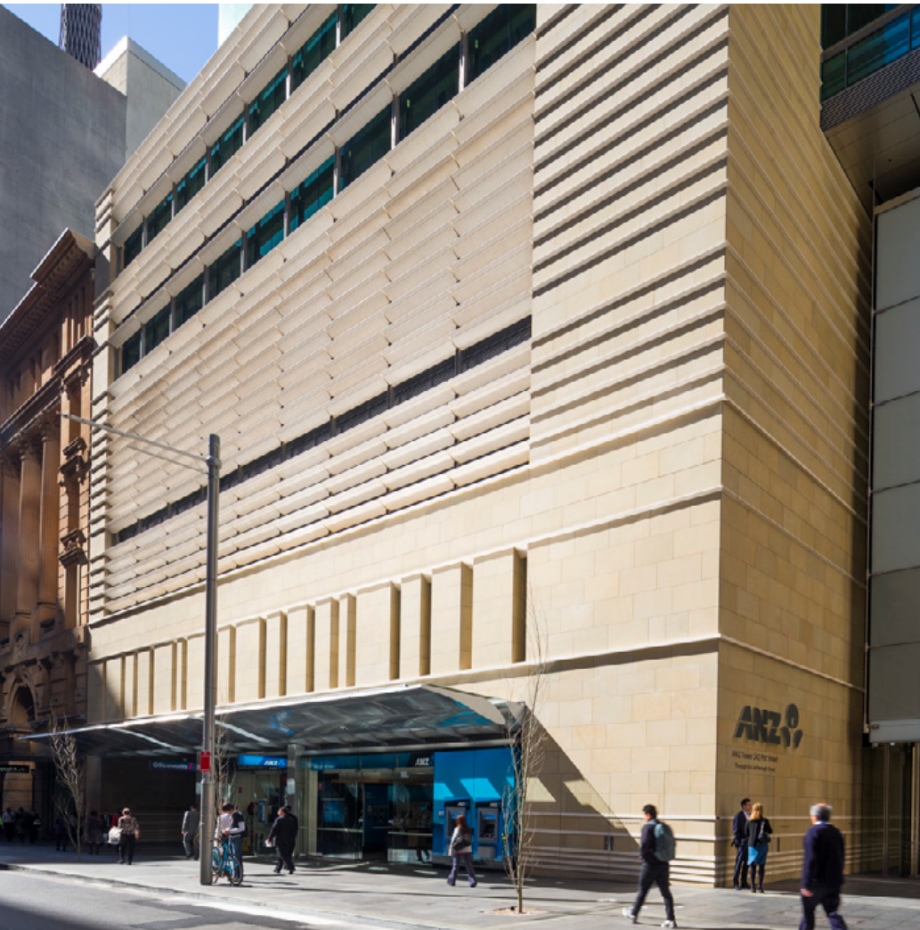
GRC Sandstone Facade at Liberty Place, 242 Pitt Street
