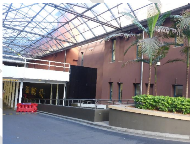
Picture 15 – Part of the eastern façade of the SELS Building.
