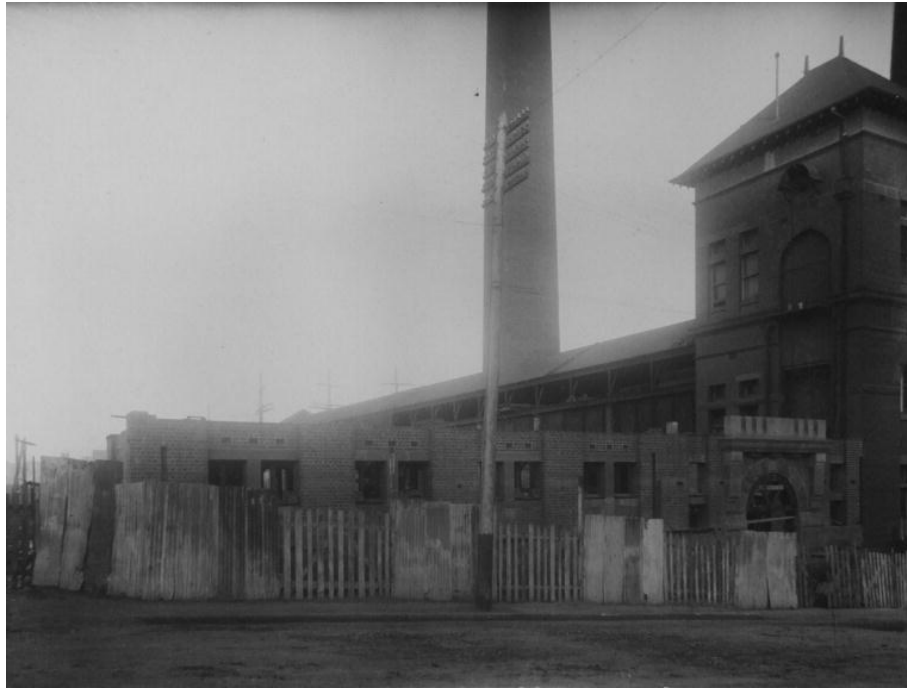
Picture 43 – October 1920. View towards the western façade.
