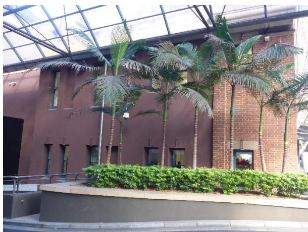
Picture 14 – Part of the eastern façade of the SELS Building.
