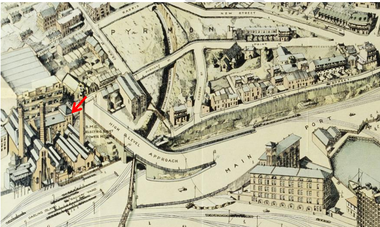
Figure 12 – Birds Eye View showing new wharves and approaches, Jones Bay, Pyrmont, c1919. The location of the subject site is indicated (and forms part of the larger power station site)
