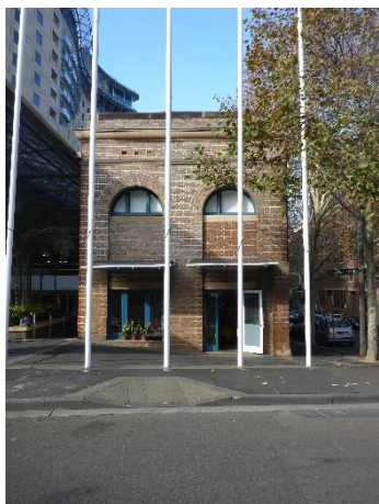
Picture 12 – Part of the northern façade of the SELS Building.
