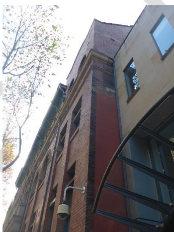
Picture 16 – Part of the southern façade of the SELS Building.
