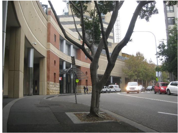
Picture 9 – View along the northern boundary of the site (Jones Bay Road).
