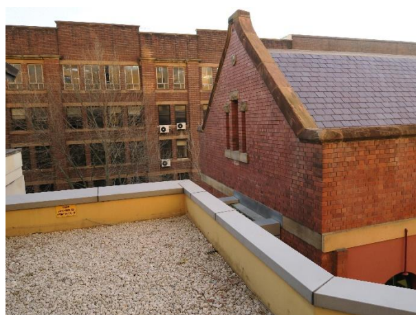
Picture 17 – Part of the eastern façade of the SELS Building.
