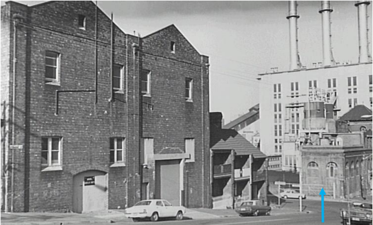
Figure 31 - C1970. Looking south east down Pymont Street from cnr of John Street. The Boilerhouse to the east of The SELS (blue arrow) had been removed by this time.
