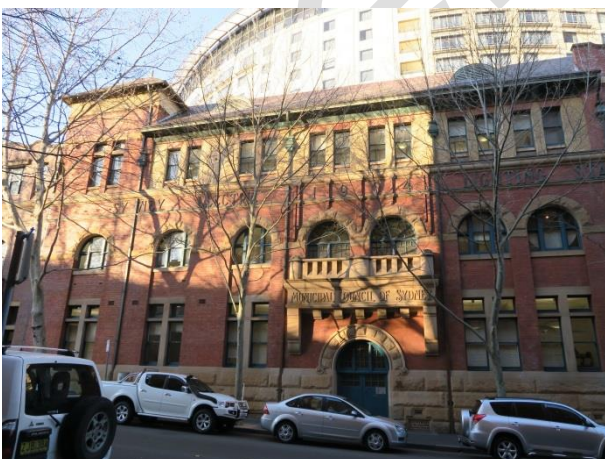
Picture 10 – Part of the western façade of the SELS Building (original 1904 Section).
