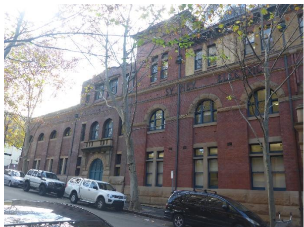
Picture 11 – Part of the western façade of the SELS Building (towards later 1920s section).
