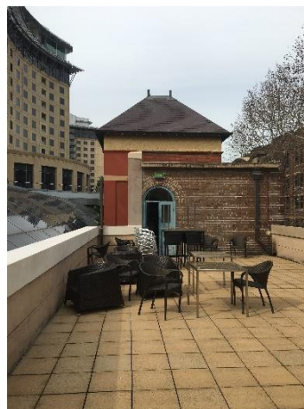
Picture 13 – Part of the eastern façade of the SELS Building.
