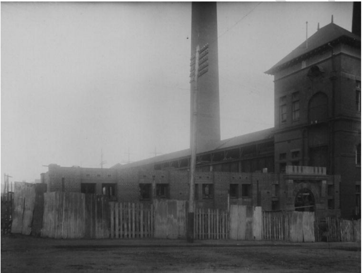
Picture 26 – October 1920. View towards the western façade.
