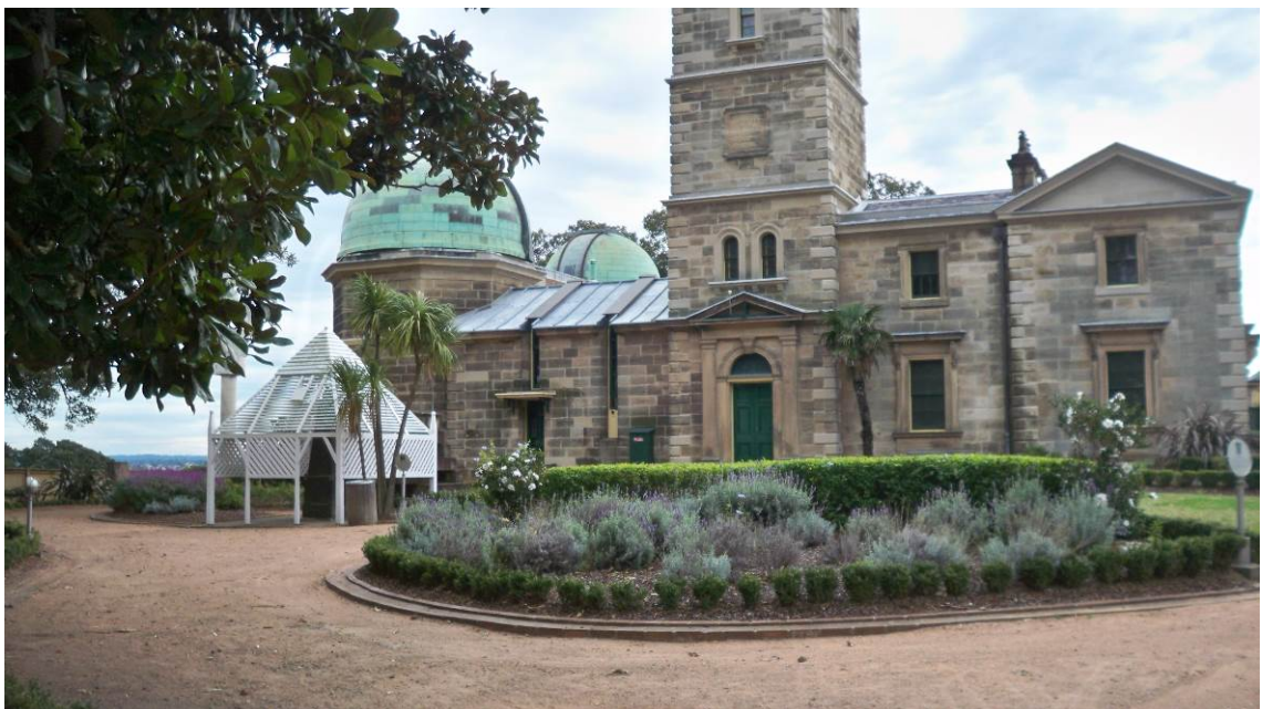
Fig 3.3 – View of South and North Domes, and courtyard, looking north
