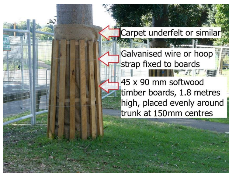
Figure 3 – Detail of Trunk Protection
