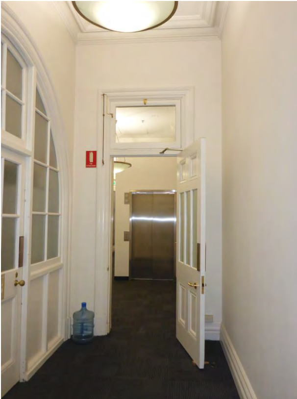
Picture 83 - First floor (Level 01) door to lift lobby has 3 panes of vertical glass to the panelled door.
