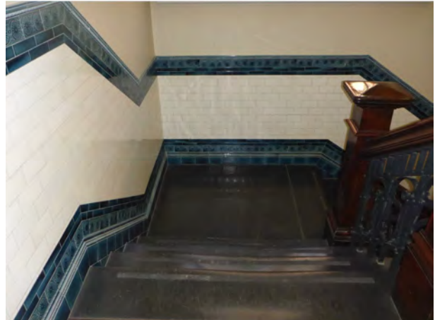
Picture 38 ĩ Stairwell view showing tiling to dado.
