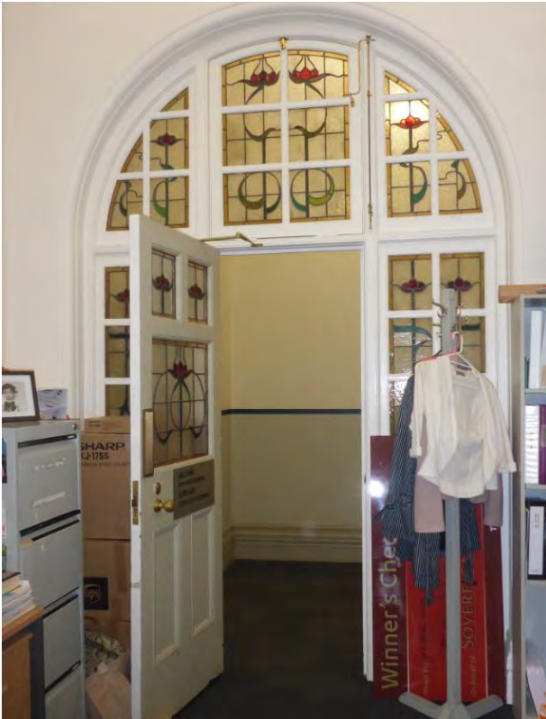
Picture 79 ĩ Typical glazed doorset with stained glass (1904).
