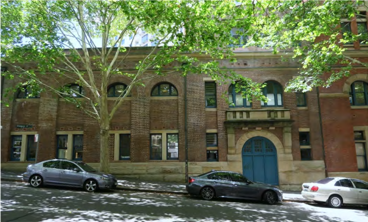
Picture 12 ĩ Western principal façade of the SELS building (1922 portion).
