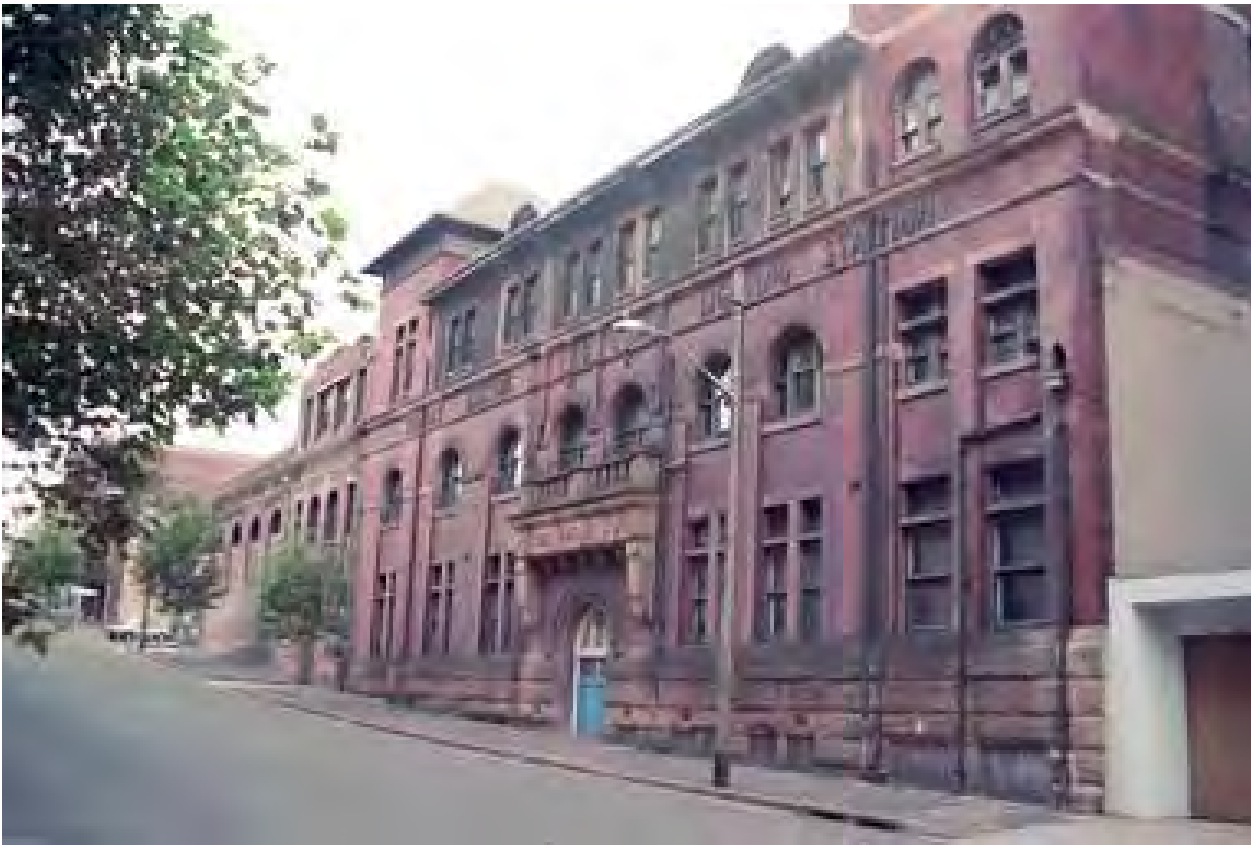
Figure 55 ĩ c1990s. Western façade of the Pymont Power Station.
