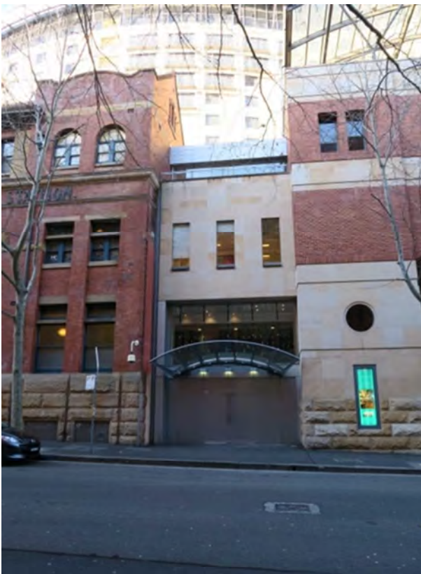
Picture 20 i View east towards the contemporary building which obscures must of the southern facade
