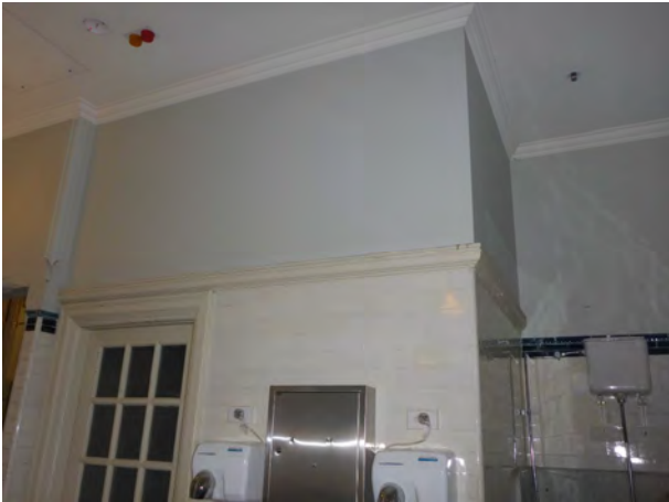
Picture 58 ĩ Original executive toilets south end of Level 01.
