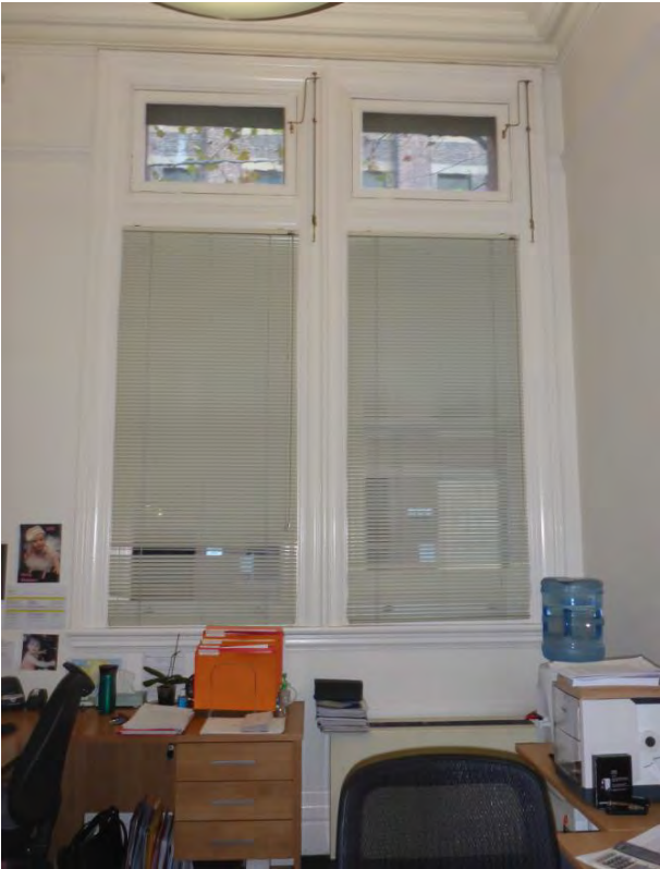
Picture 71 ĩ Typical Paired Windows in East Façade.
