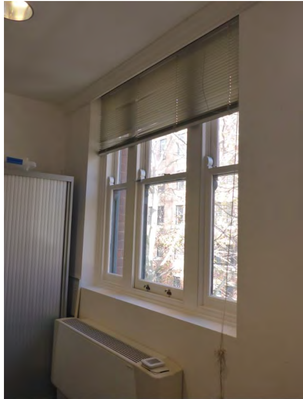
Picture 76 - Windows on Second Floor Space 02/03.
