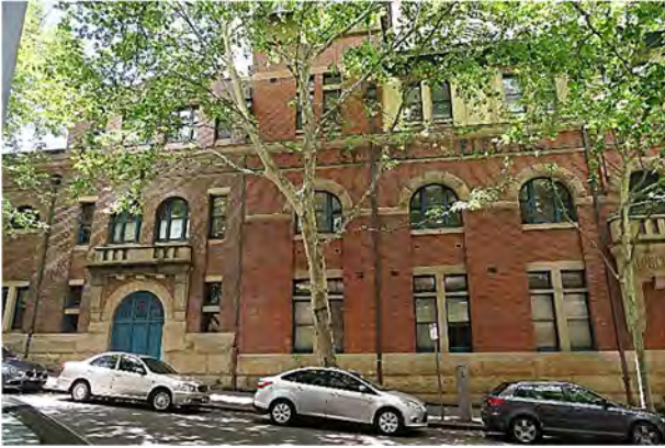
Picture 7 ĩ Streetscape view to part of the western façade from the west.
