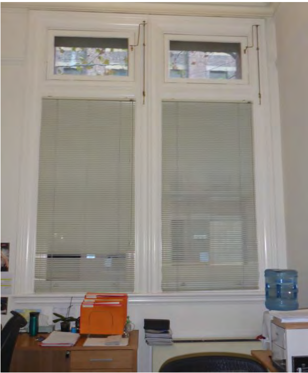
Picture 73 ĩ Typical interior view of a paired large window on the main façade showing architraves and sill.
