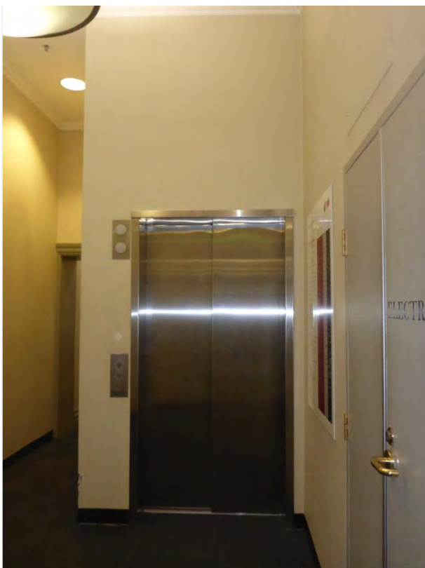
Picture 89 i External view of c1995 elevator. Ground Floor.
