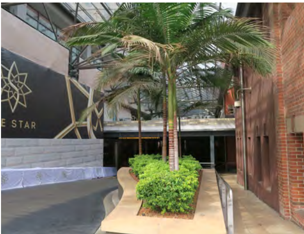
Picture 26 ĩ View south along the eastern façade of the SELS.
