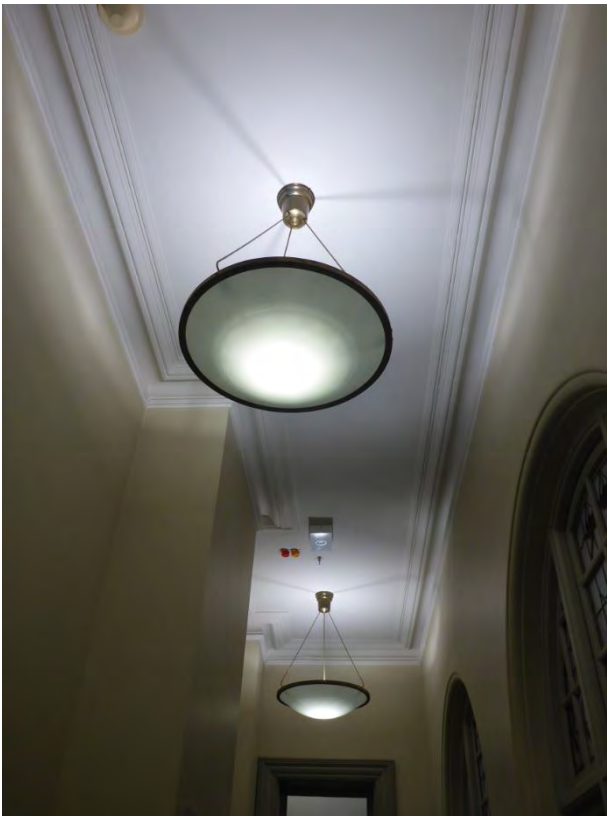
Picture 66 Ĩ Typical plaster ceiling and cornice to the main corridor.
