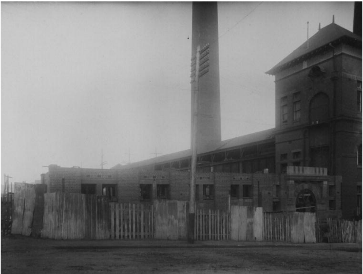
Picture 98 ĩ October 1920. View towards the western façade
