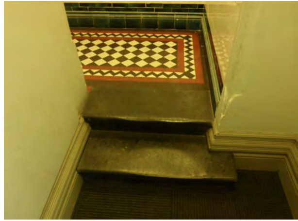
Picture 59 ĩ Original Executive toilets south end of Level 01.
