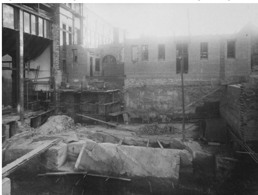
Figure 66 - c1903 Original Southern elevation of the building showing the abutting building to the rear (east).
