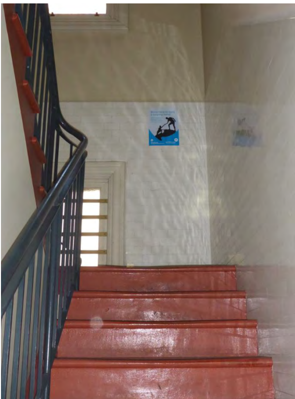
Picture 60 ĩ Secondary (northern) staircase.
