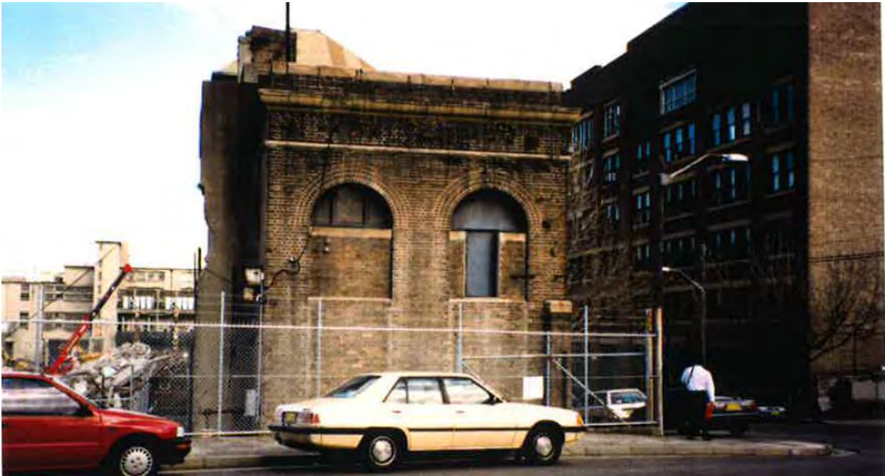
Picture 109 Ĩ North elevation of the Offices of the Sydney Electric Lighting Station Source: Conservation Management Plan (Tanner) 1994
