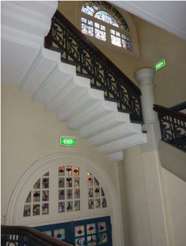
Picture 32 ĩ Main Stairwell view from Level 00 landing.
