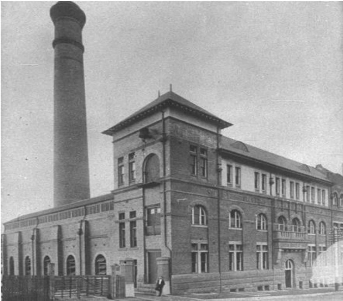
Figure 46 ĩ c1905. Northern extent of the original 1904 section of the Sydney Electric Lighting StationòPowerhouseĭ Pyrmont
