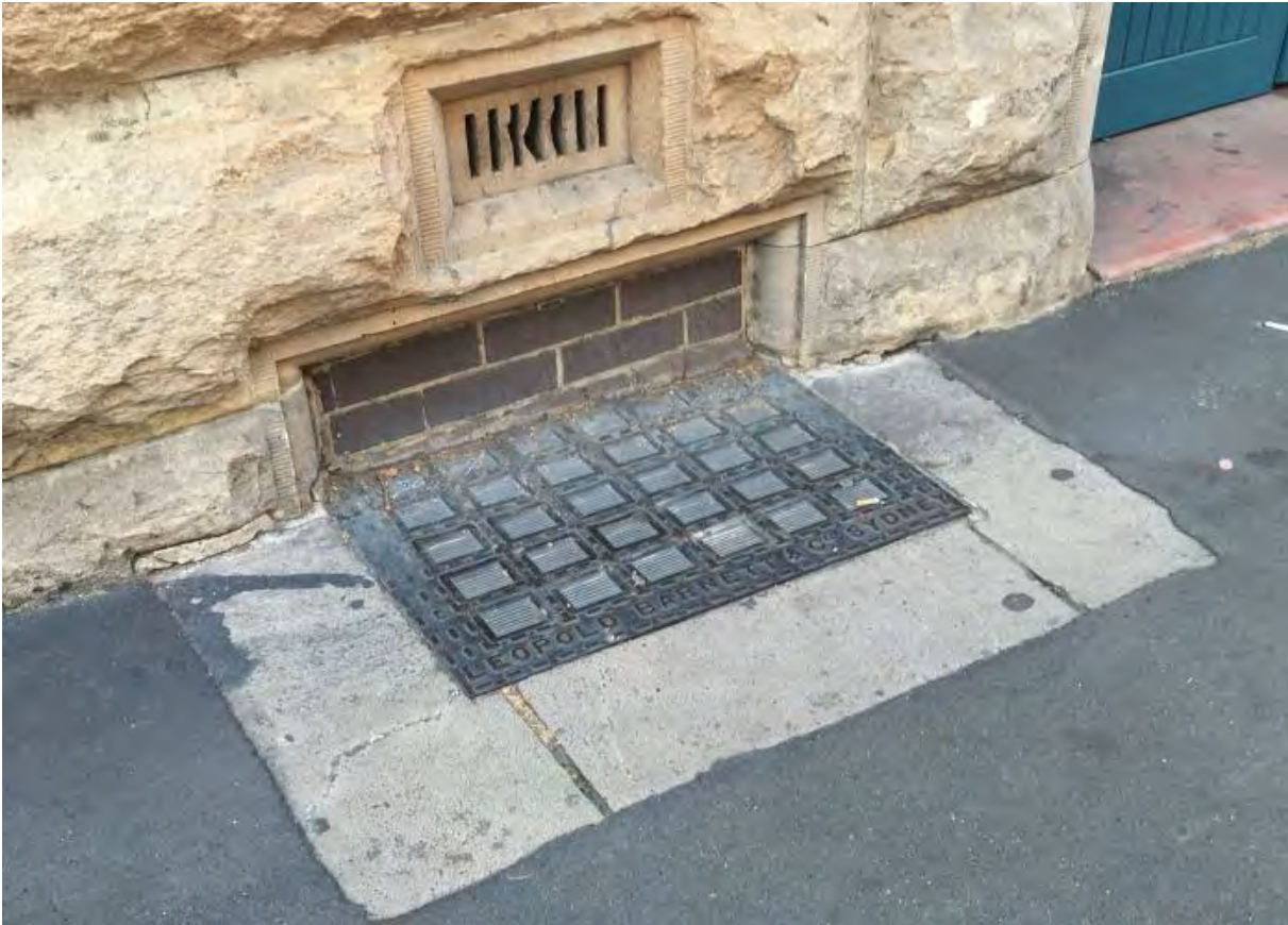
Picture 14 ĩ Pavement light (detail).
