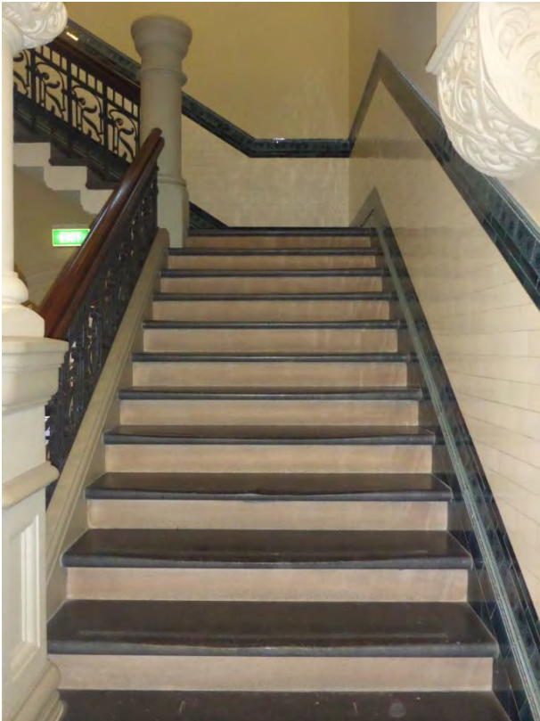
Picture 35 ĩ Typical stair flight with tiled dado.
