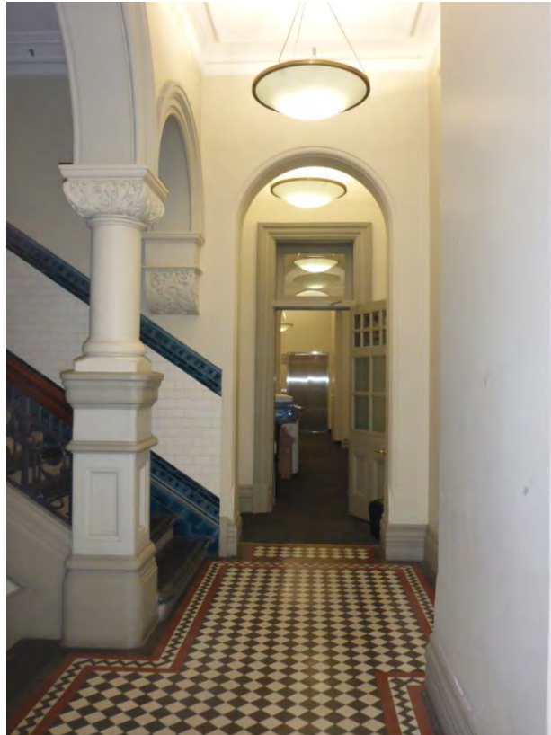
Picture 31 i Main Stairwell Landing at level 00 (Ground).
