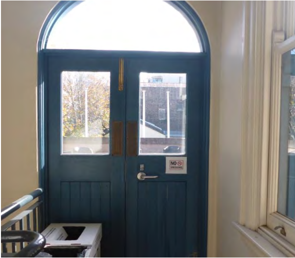
Picture 18 i Door onto terrace from the Northern Secondary Stair.
