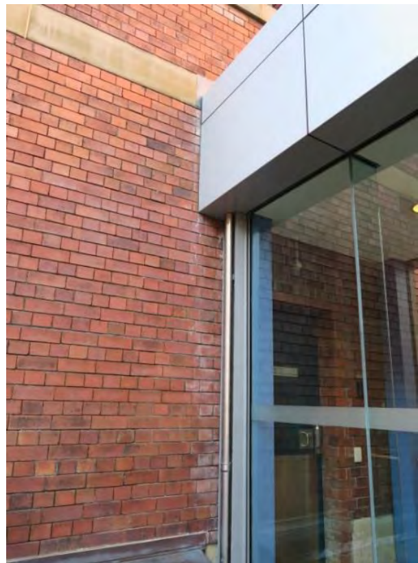
Picture 21 i View of the junction between The SELS and the contemporary structure adjacent, which has externalised part of the southern façade of The SELS.
