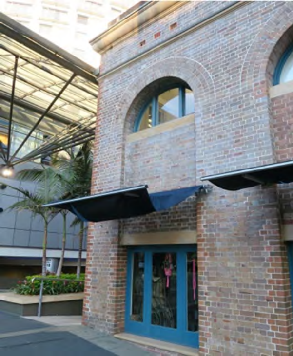
Picture 25 ĩ Part of the northern façade of the SELS Building showing later opening and awning to the ground floor.
