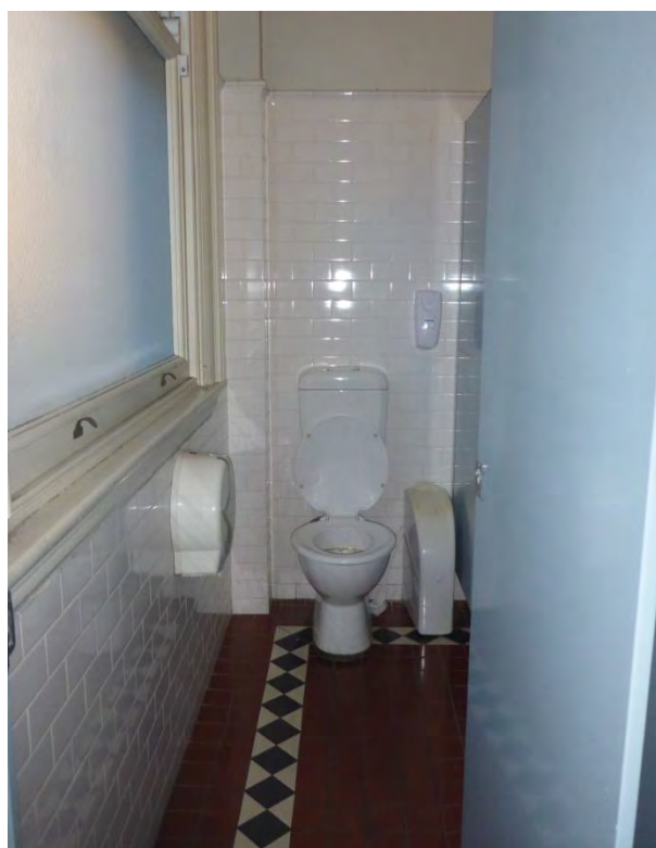
Picture 53 i Later fitout to the ground floor bathroom. Tiling is c1996.
