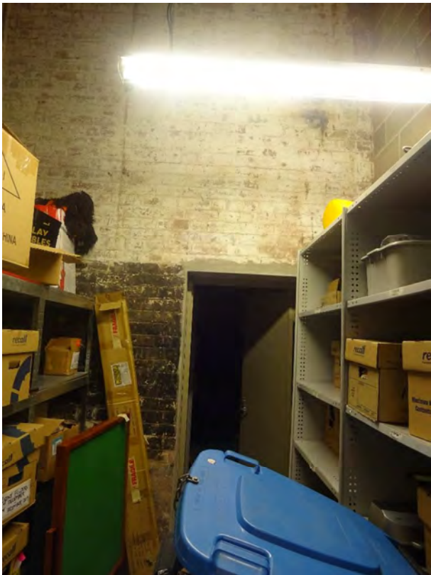
Picture 92 ĩ View of basement.
