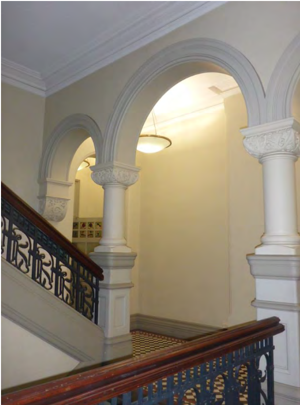
Picture 30 i Main Stairwell Landing at Level 00 (Ground).
