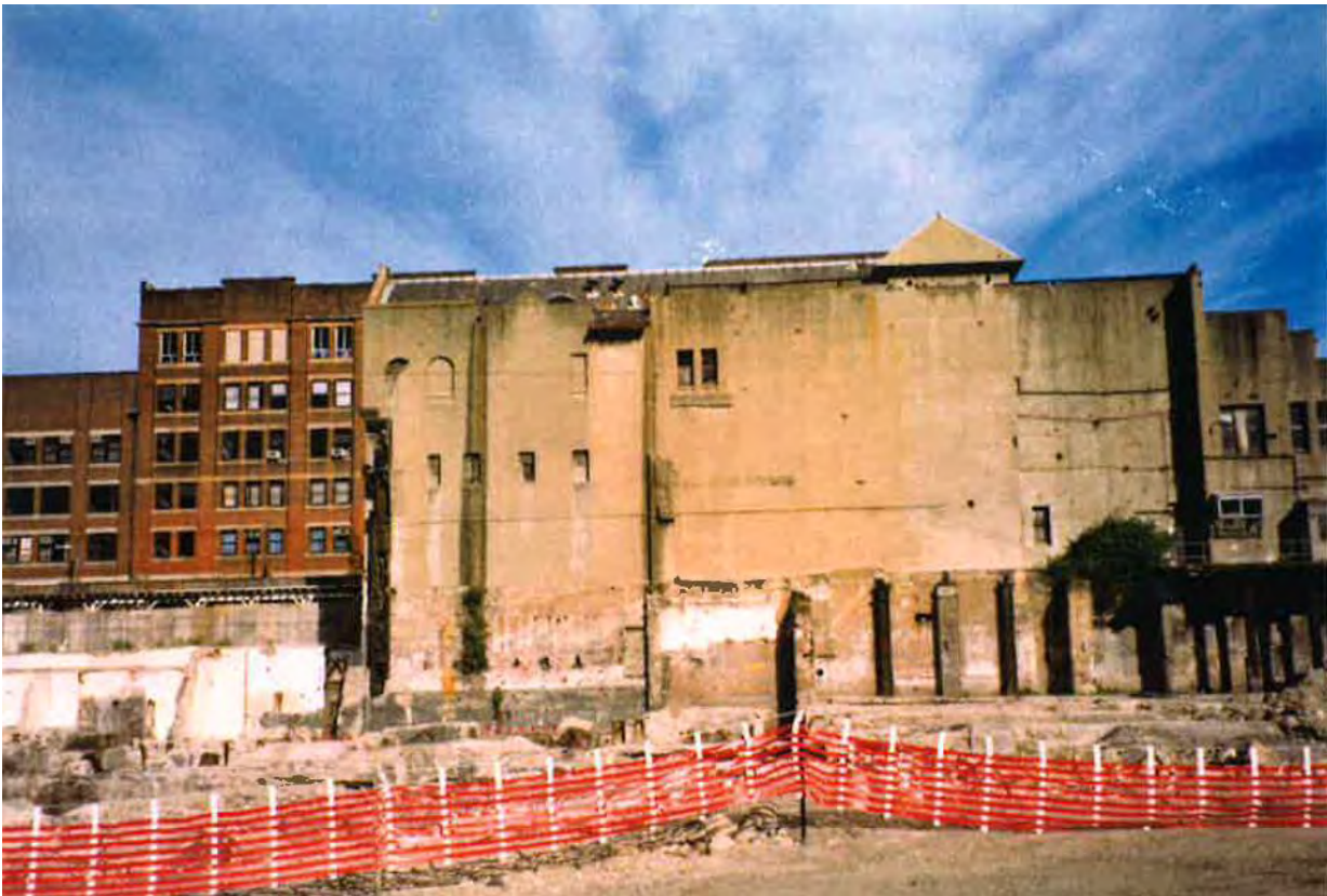
Picture 107 ĩ East elevation of the offices of the Sydney Electric Lighting Station Source: Conservation Management Plan (Tanner) 1994
