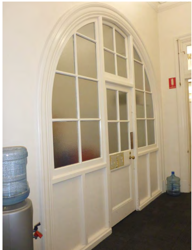
Picture 86 i First Floor (Level 01) (door to 01/11 from corridor 01/04).
