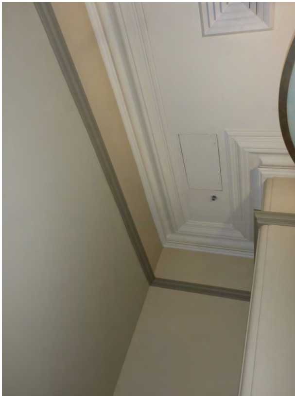
Picture 67 Ĩ Typical plaster ceiling and cornice.
