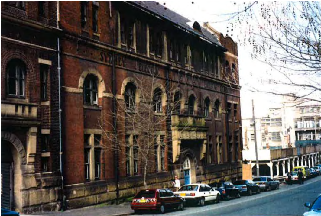
Picture 108 ĩ West elevation to Pymont Street Source: Conservation Management Plan (Tanner) 1994
