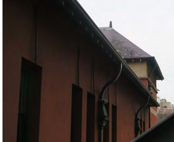
Picture 23 ĩ View over the roof eaves and tower form the west.
