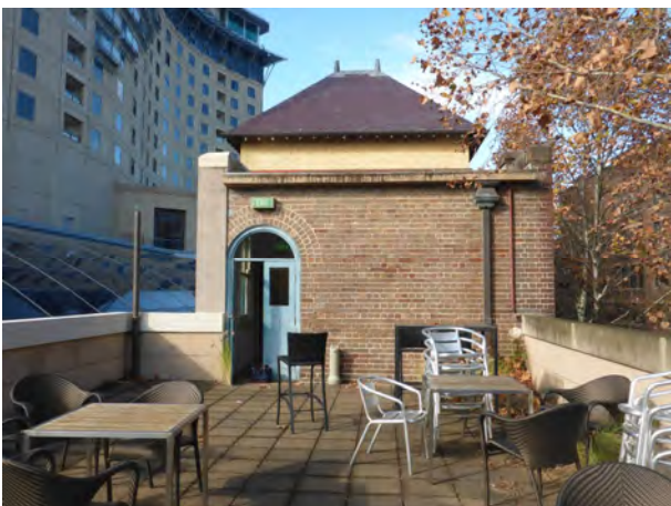
Picture 16 ĩ Second Floor North elevation onto terrace.
