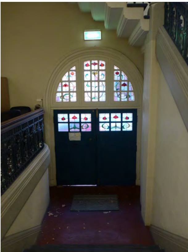
Picture 34 ĩ Main Stairwell view to original front door at level 00.
