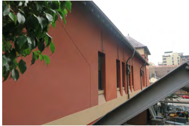
Picture 29 ĩ View towards the eastern façade of the SELS, second floor.
