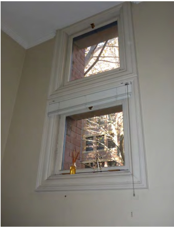
Picture 74 ĩ Typical interior view of a smaller window on the main façade showing architraves and lack of articulated sill.
