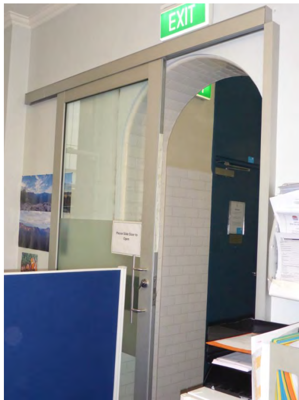
Picture 61 ĩ Doorway into the second (northern) staircase from the ground floor corridor.
