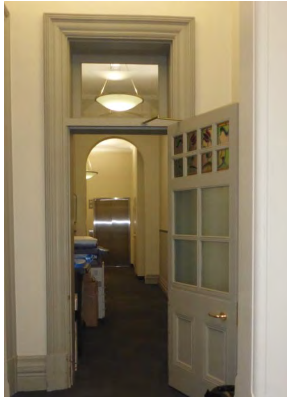
Picture 80 ĩ Door with half glazing and some leadlight to Corridor Level 00 (Ground) leading north from main stairwell.
