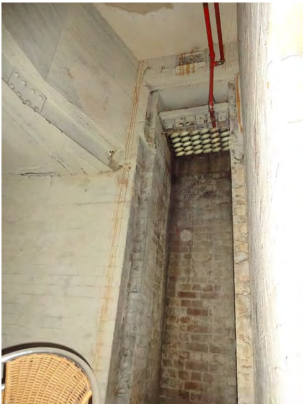
Picture 93 ĩ Image showing underside of pavement light.
