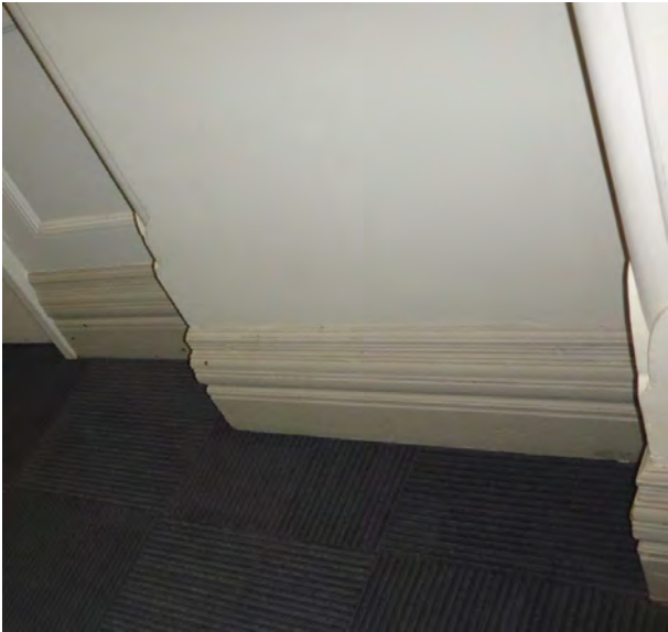
Picture 87 i Typical Skirting Boards.
