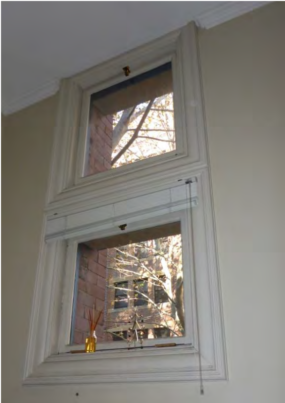
Picture 72 ĩ Typical small windows in East façade office.
