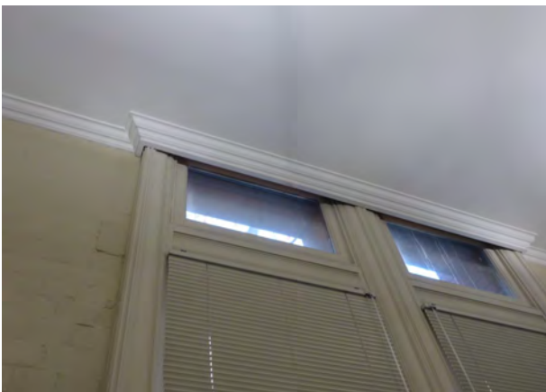
Picture 77 i Typical recent false ceilings obscuring the top of the windows.
