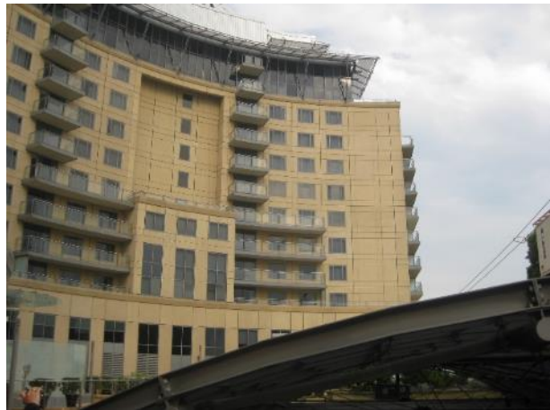
Picture 5 Ĩ View west towards the Astral Tower.
