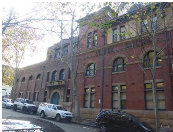
Picture 11 i Part of the western façade of The SELS Building (towards later 1920s section).
