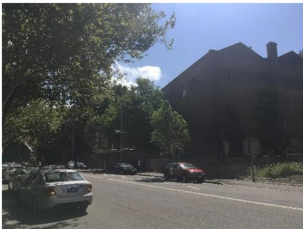
Picture 22 i View west towards the Slades Warehouse Building.
