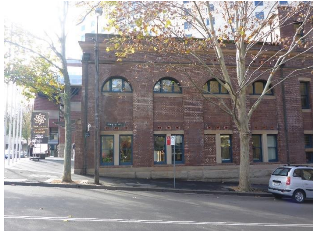
Picture 56 ĩ View west from the corner of Harris Street and Scott Street
