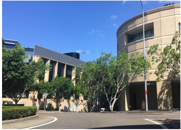
Picture 40 ĩ View east towards the existing development on the north corner of the subject site.
