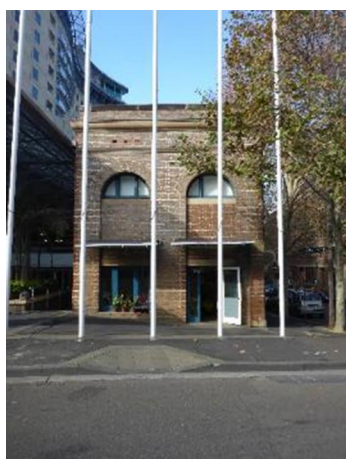
Picture 12 i Part of the northern façade of The SELS Building (towards later 1920s section).
