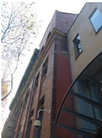
Picture 16 ĩ Part of the southern façade of The SELS Building.
