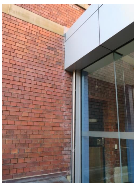
Picture 10 Ĩ View of the junction between The SELS and the contemporary structure adjacent, which has externalised part of the southern façade of The SELS.
