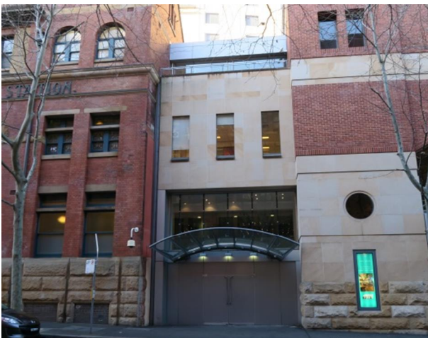
Picture 3 ĩ Western façade showing the relationship between the southern façade and the contemporary building to the south of the SELS.
