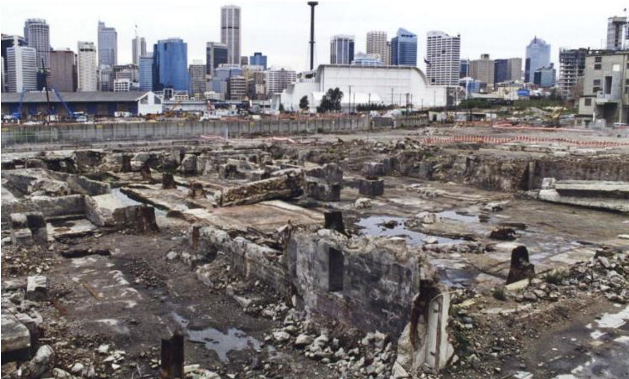
Picture 20 i View of the site, facing east
