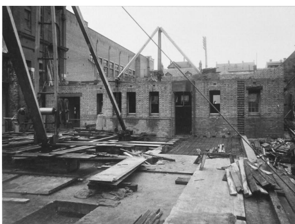
Picture 7 Ĩ 1921. View west towards the eastern façade of The SELS under construction.
