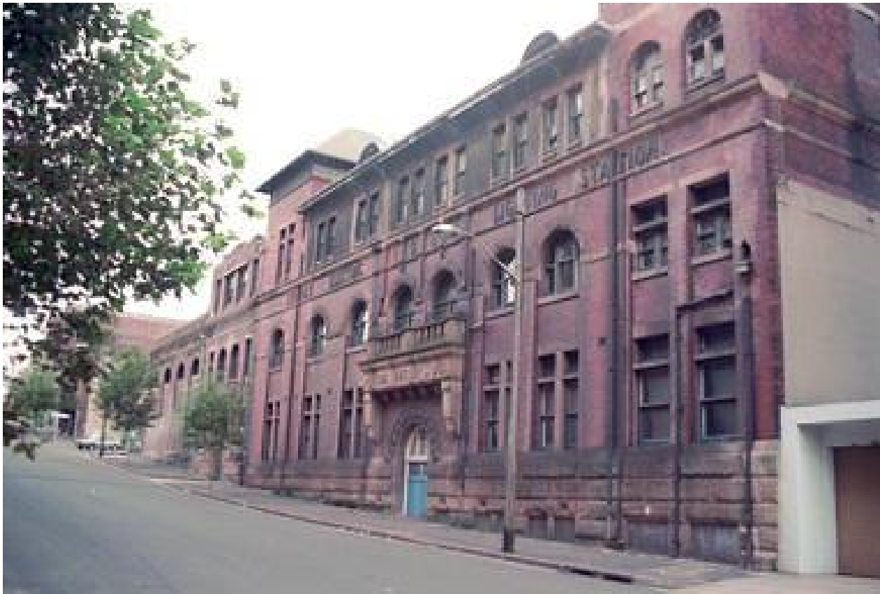
Figure 26 ĩ c. 1990s. Western façade of the SELS building, retained on site
