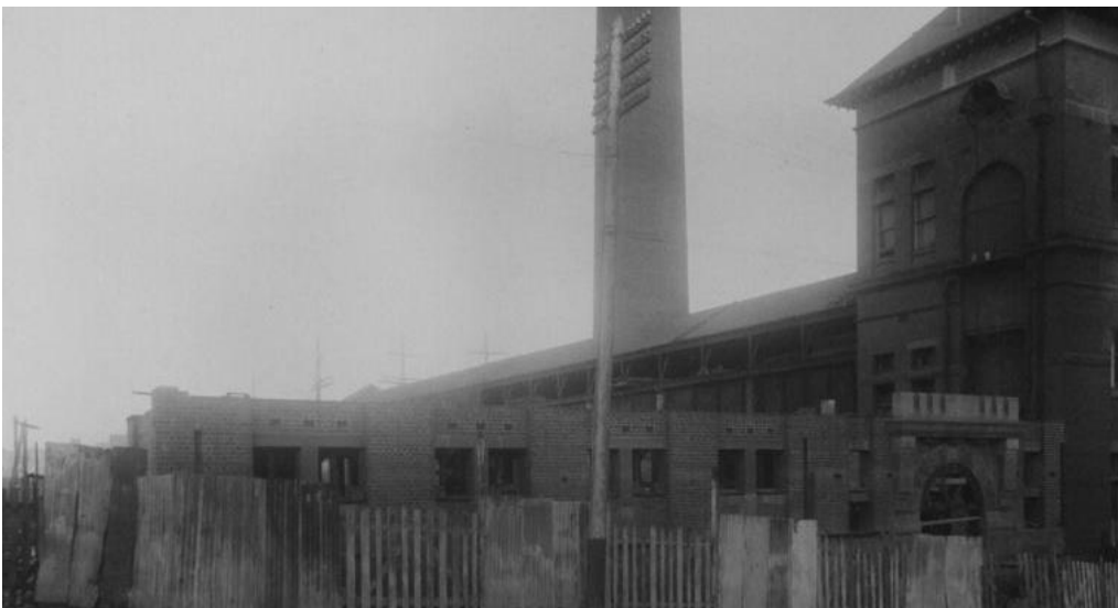
Picture 17 Ĩ October 1920. View towards the western façade.
