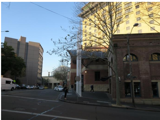
Picture 5 Ĩ View north east up Jones Bay Road.
