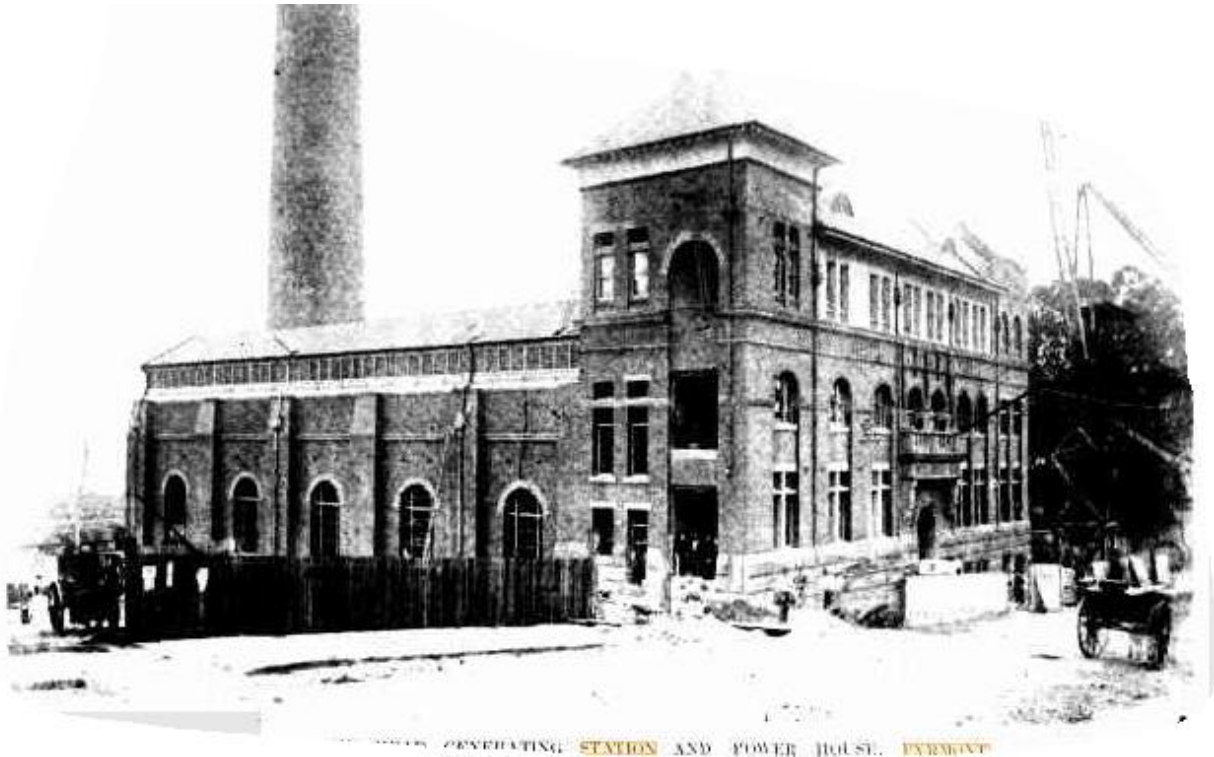
Figure 13 ĩ The opening of the head Generating Station and Power House, Pyrmont. Note SELS Building fronting Pyrmont Street.
