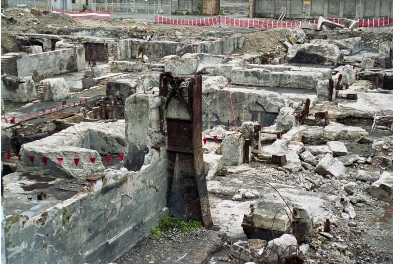
Picture 19 i View of the site
