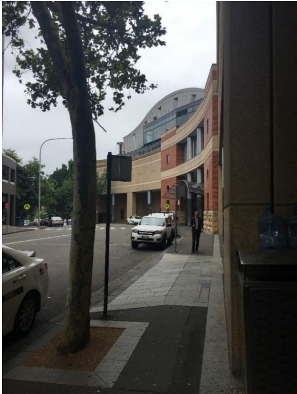
Figure 9: North western face, Jones Bay Road, looking north (February 2017)
