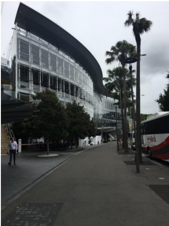
Figure 8: the eastern façade of The Star – The Ribbon facing Pyrmont Bay, facing west, Pirrama Road (February 2017)
