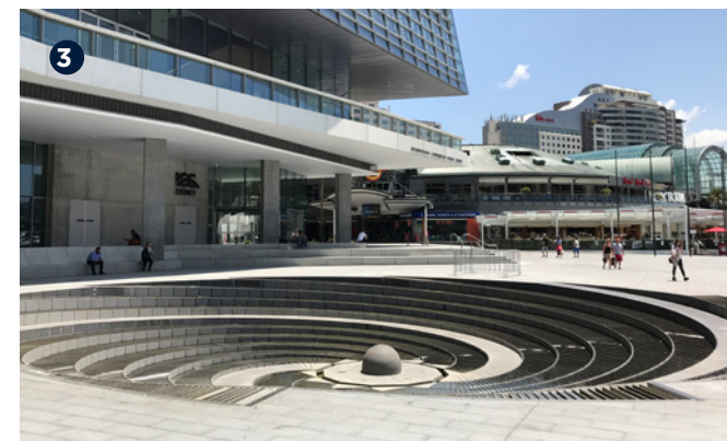
Renovated water feature at ICC entry
