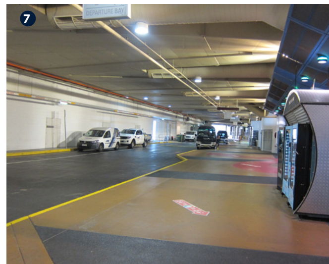
Port Cochere besides Light Rail
