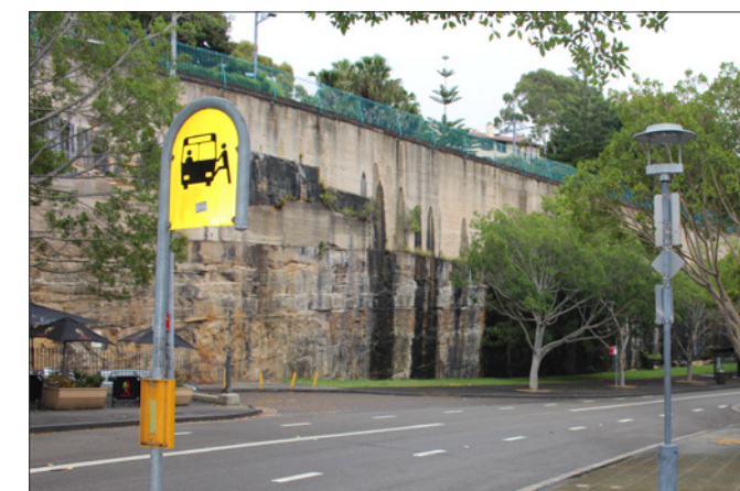
FIGURE 26: Photo A of existing sandstone cliffs
