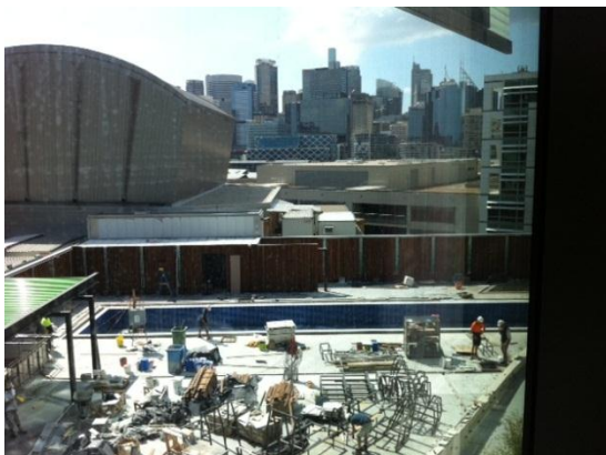
PICTURE 1 – VIEW OF POOL DECK TO NORTH-EAST
