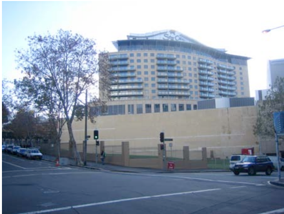
Picture 1 – The 'Switching Station' site (vacant foreground)
