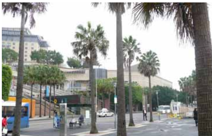
PHOTOS LOOKING SOUTH (ABOVE) AND NORTH (BELOW) ALONG PIRRAMA ROAD. THE PODIUM IS HARDLY VISIBLE LOOKING SOUTH, WITH INCREASED VISIBILITY LOOKING NORTH. THE PROPOSAL WILL CONTINUE THE EXISTING SCALE OF THE PODIUM ALONG PIRRAMA ROAD, THE NEW TOWER WILL BE VISIBLE CLOSE TO THE SITE LOOKING SOUTH WEST BALANCING THE EXISTING TOWER VISIBLE IN THE CENTRAL PHOTO
