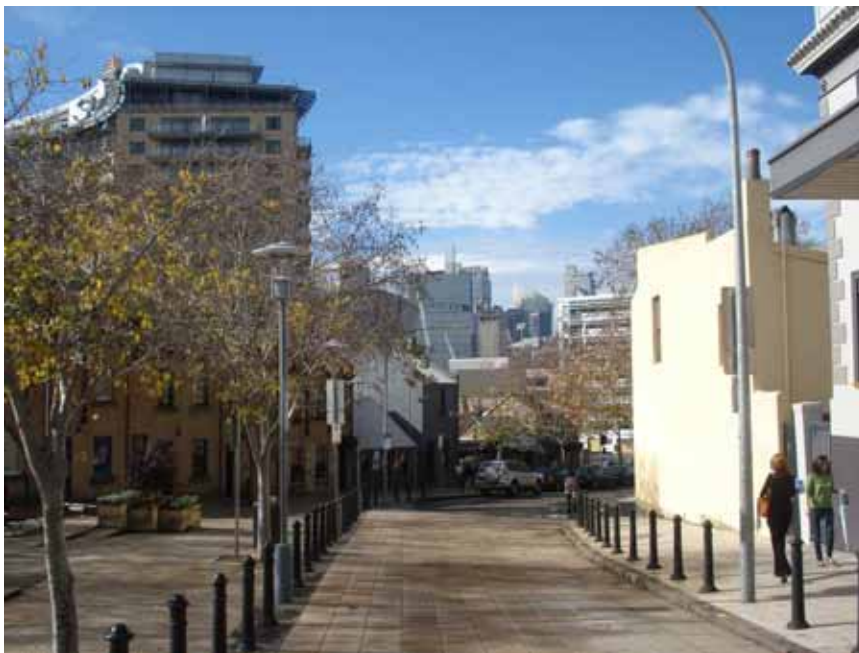
PHOTO FROM THE SOUTHERN SHAREWAY LOOKING TOWARDS THE NORTH WEST CORNER OF THE INTERSECTION OF PYRMONT AND UNION STREET. THE PODIUM WILL BE BARELY VISIBLE, THE TOWER FORM WILL BE STRONGLY VISIBLE AND WILL INFILL THE MAJORITY OF THE SKYLINE FROM THIS VIEWPOINT TO A HEIGHT EQUIVALENT TO THE EXISTING CASINO TOWER
