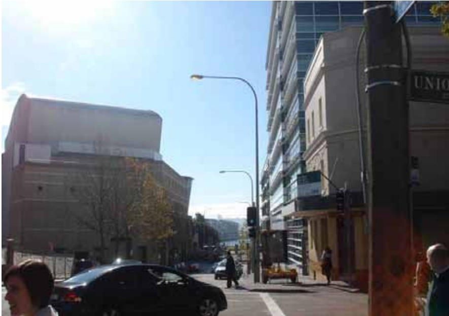
PHOTOGRAPH LOOKING DOWN EDWARD STREET TOWARDS THE WATER AND PIRRAMA ROAD SHOWING THE GREATER SCALE TO THE EAST AND THE EXISTING PODIUM FORM AND LYRIC THEATRE TO THE LEFT HAND SIDE OF THE IMAGE
