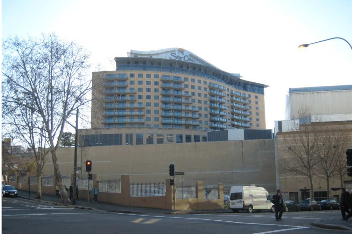
Figure 3 – Existing Star City Complex with Switching Station site in foreground
