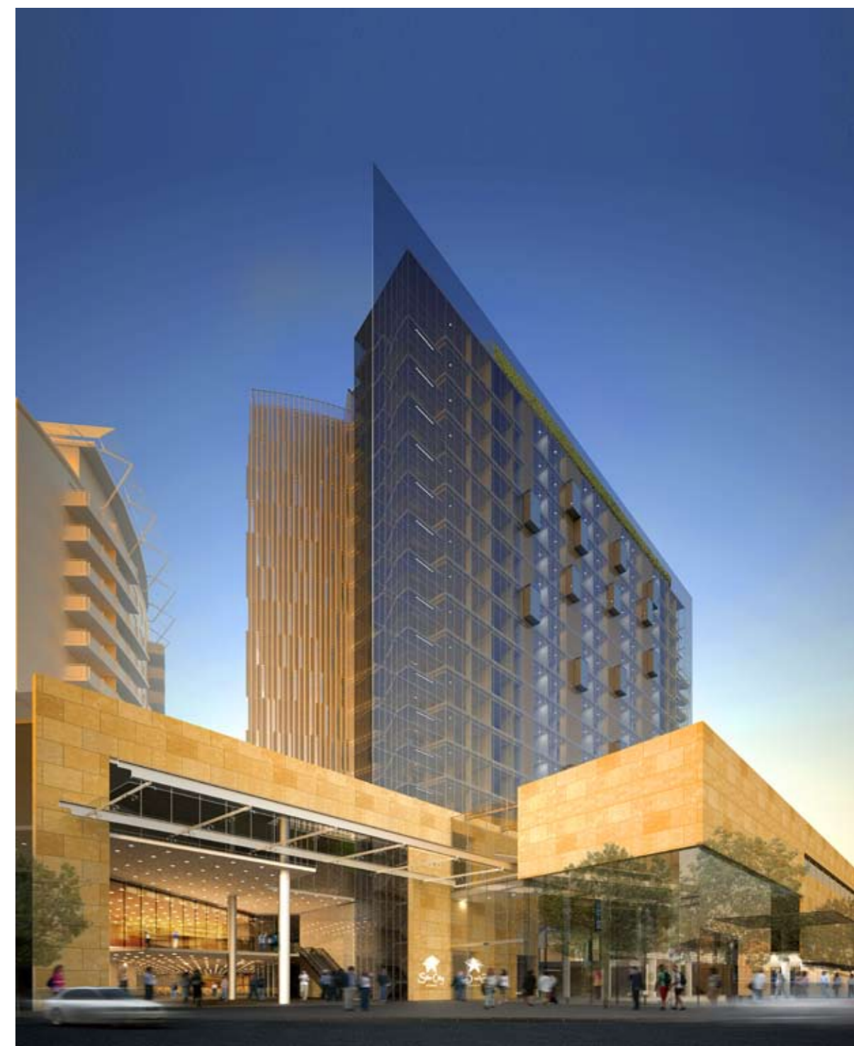
Union / Pyrmont Street Entry
