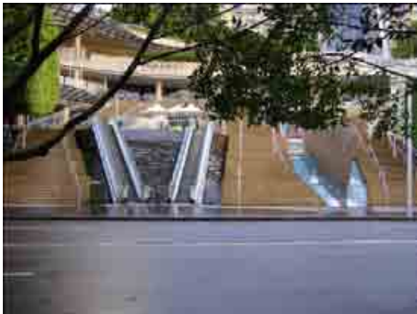
Picture 5 – Existing Pirrama Road Stairs
