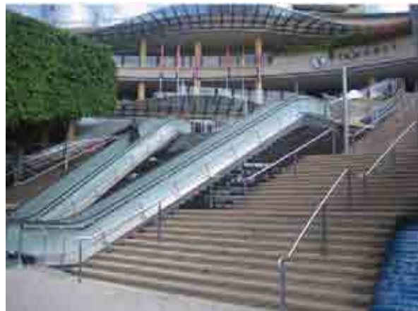
Picture 6 – Existing Pirrama Road Stairs
