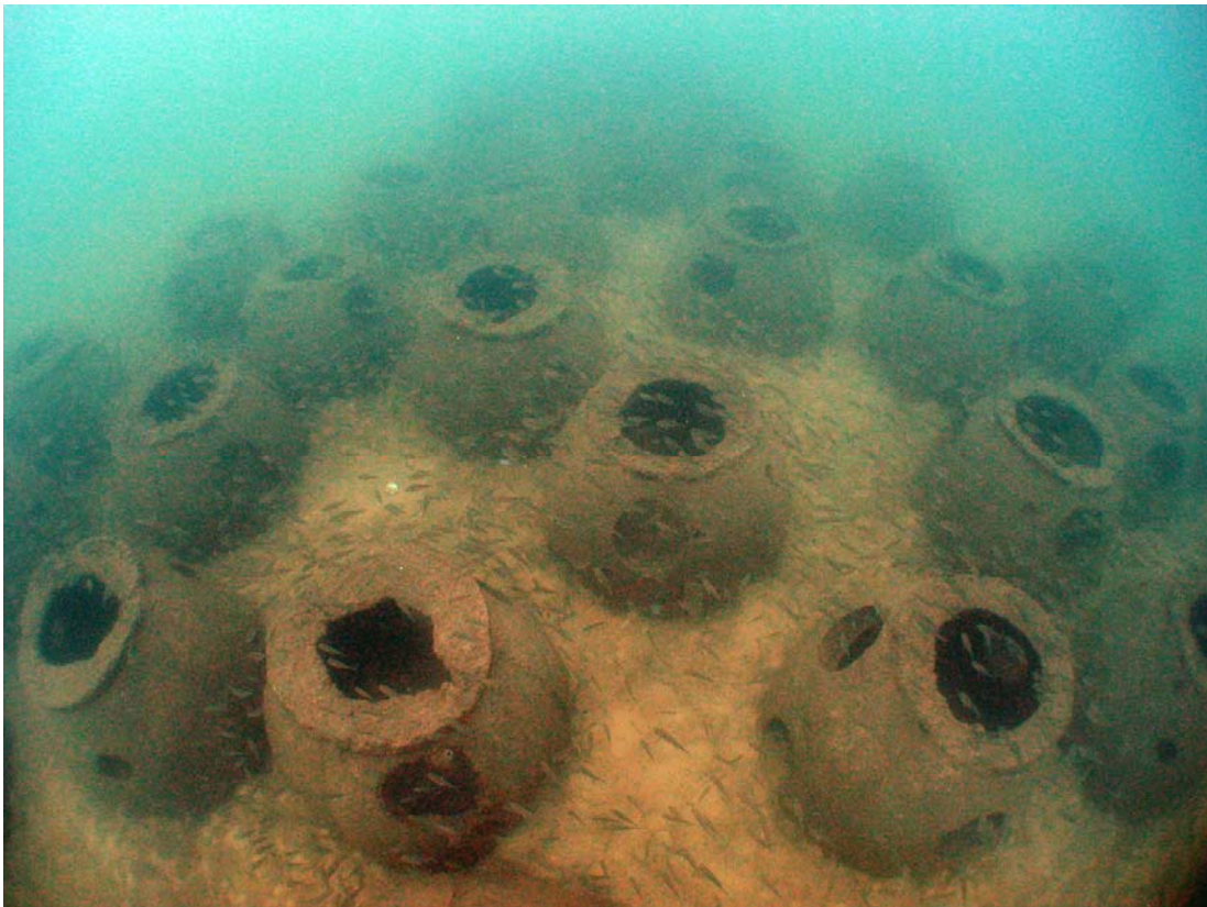
Figure 3: Individual concrete 'Reef Ball' artificial reef units deployed together in Lake Macquarie in December 2005 form a reef group (image: NSW DPI).
