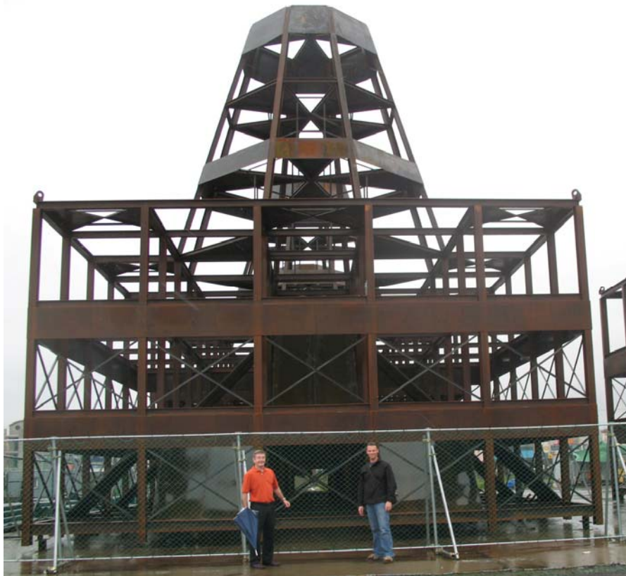
Figure 6: A 10 m tall, 35 tonne design specific steel artificial reef unit waiting for deployment on Cheju Island, South Korea (image: NSW DPI).
