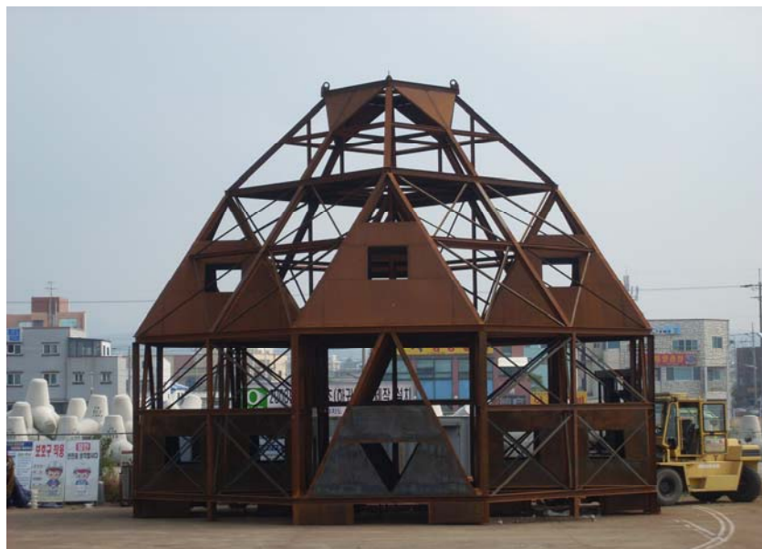
Figure 3: Examples of individual offshore artificial reef units deployed in Korea. The dimensions of the units are 13.6 m x 11 m x 11m (height, length and width) and 10 m x 12 m x 12 m (height, length and width) in (a) and (b) respectively.
