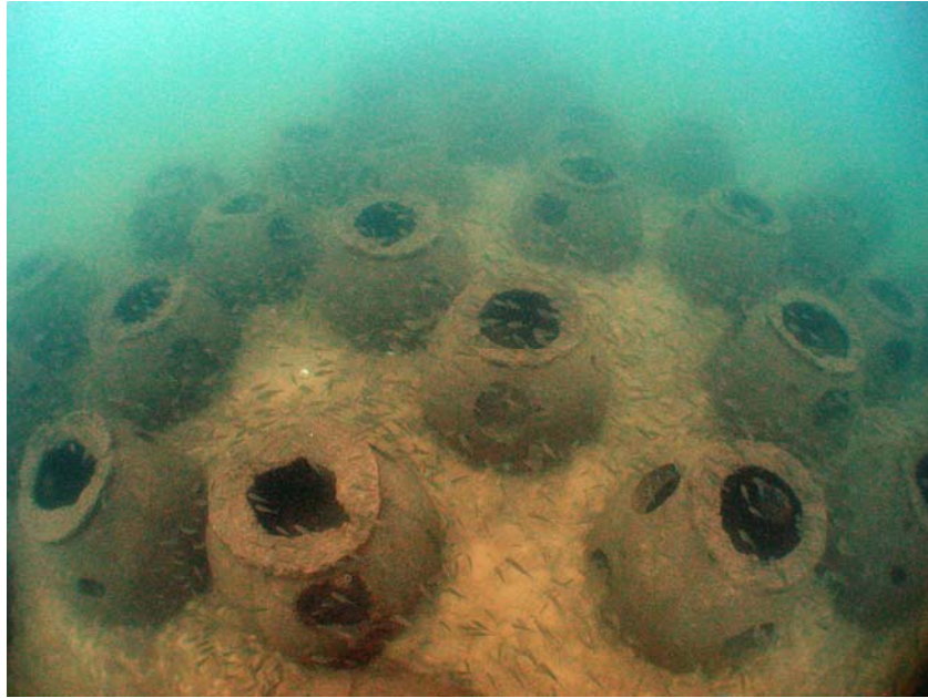
Figure 1: A collection of individual concrete Reef Balls used to create the artificial reef in Lake Macquarie in December 2005 (image: DPI)
