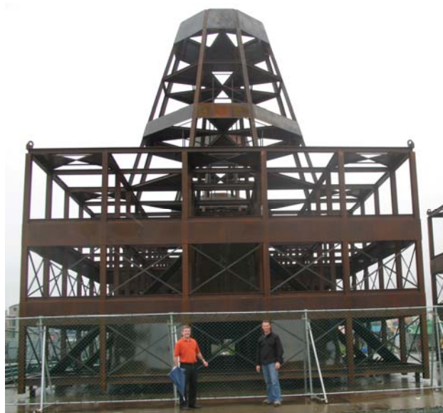
Figure 2: A completed octagonal two storied steel artificial reef unit manufactured on Cheju Island (South Korea) waiting for deployment in September 2007 (image: DPI).
