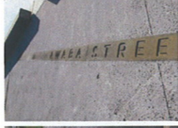
CONCRETE FLUSH EDGE Width of edge varies. Edges to be precast or insitu. Precast edges include text cast in
