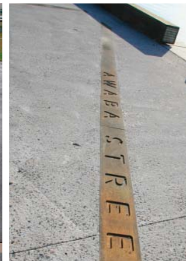
CONCRETE FLUSH EDGE Width of edge varies. Edges to be precast or insitu. Precast edges include text cast in
