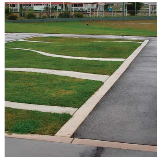
CONCRETE FLUSH EDGE Width of edge varies. Edges to be precast or insitu. Precast edges include text cast in
