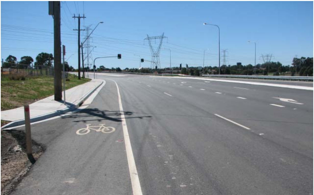
View looking north-east along Erskine park Road towards Lenore Drive.
