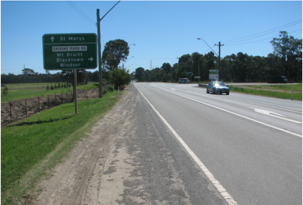
View looking north along Mamre Road on approach to Erskine Park Road.
