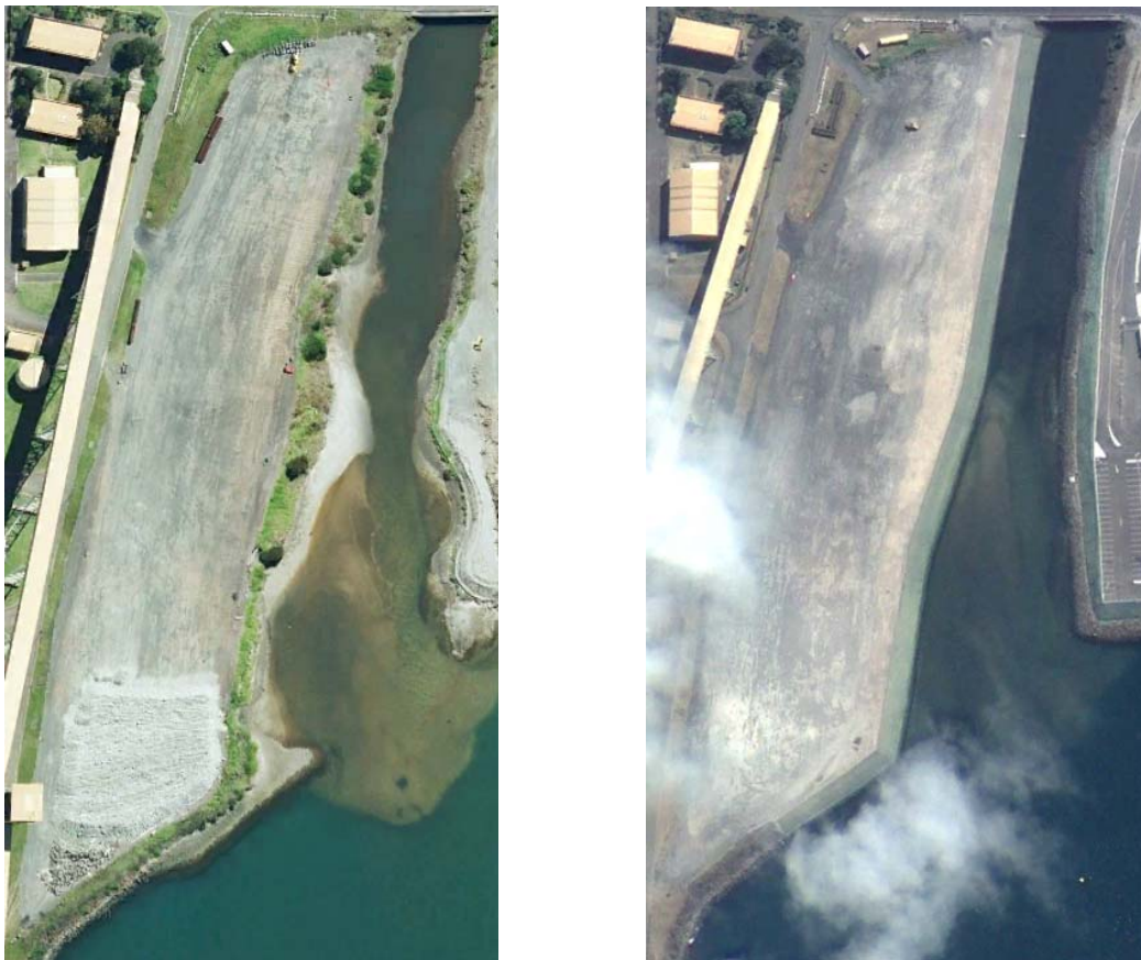
Figure 1: Allotment 5 before and after embankment stabilisation works conducted in 2009
