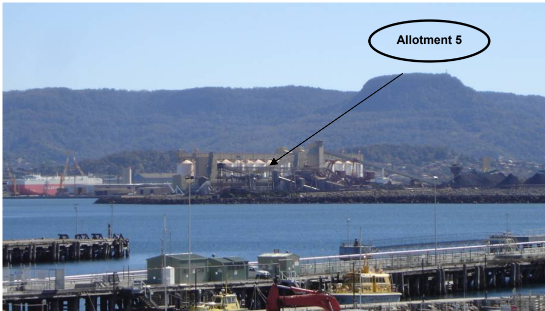
Figure 71 Viewpoint (3) from Breakwater Battery looking north-west toward subject site
