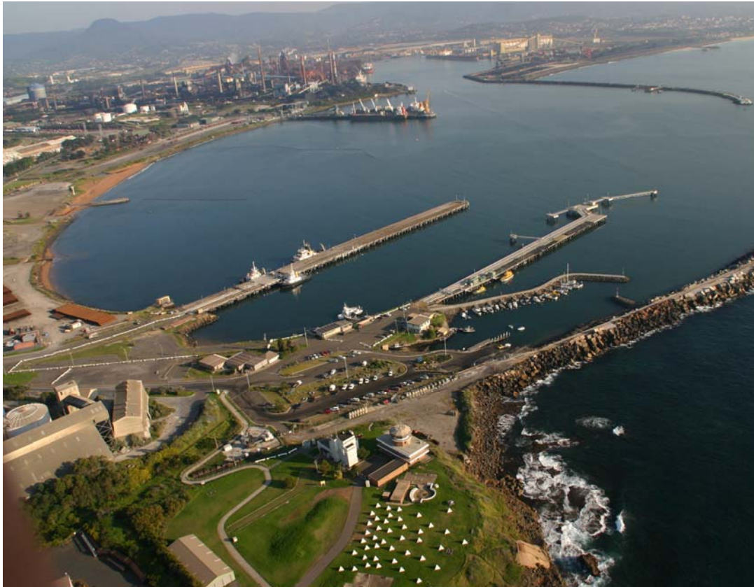
Figure 66 Looking north-west from the Outer Harbour to the Inner Harbour June 2008
