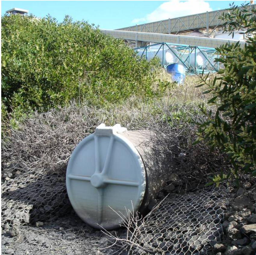
Figure 78 Stormwater outlet into the Garungaty Waterway
