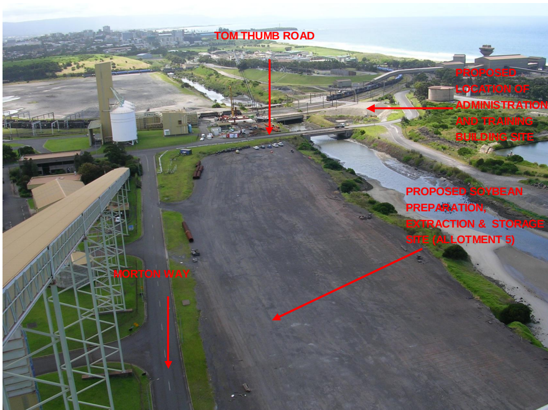
Figure 7 Allotment 5 looking north to Tom Thumb Road from GrainCorp observation tower
