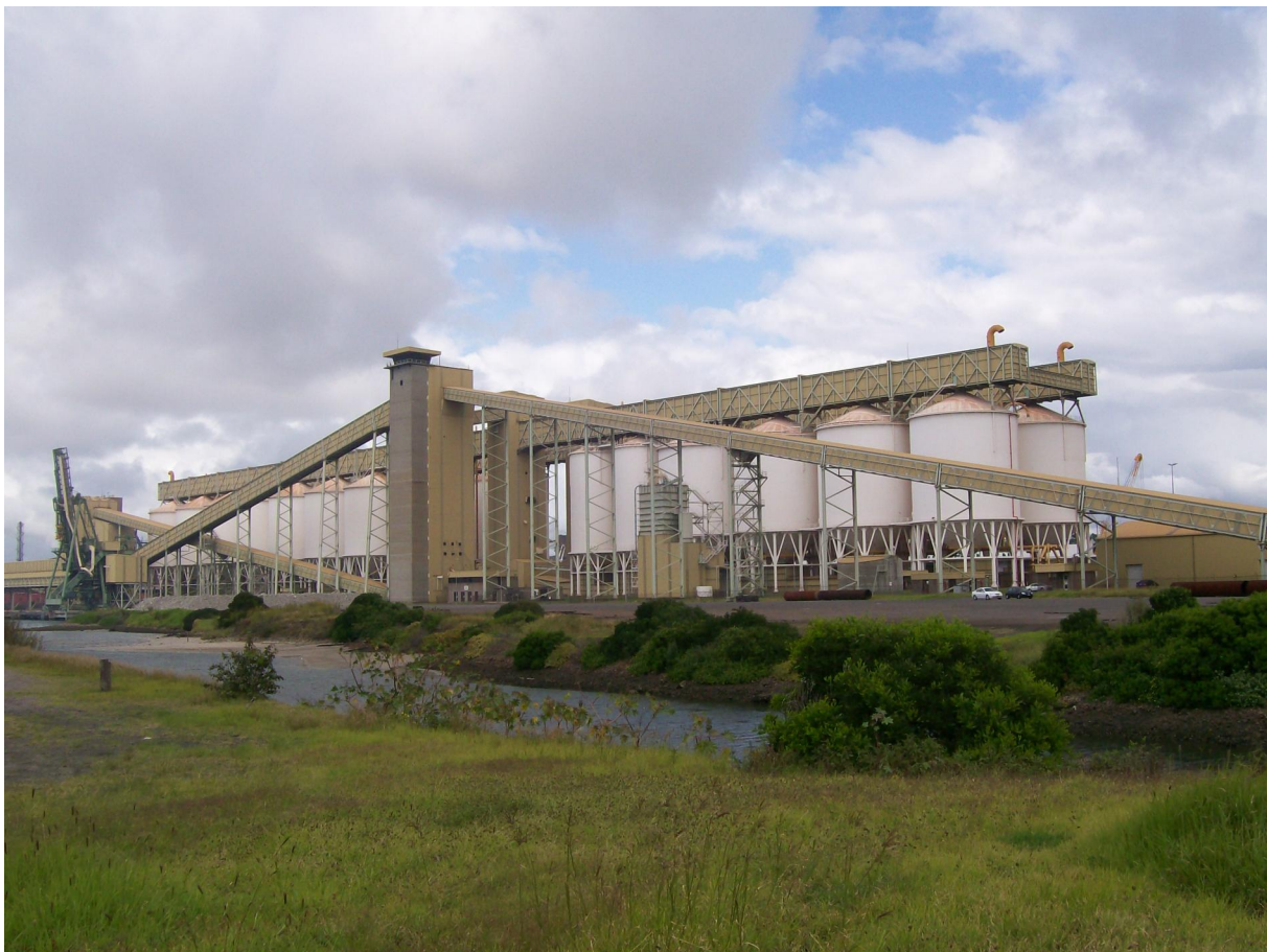
Figure 14 Land uses (Grain Terminal) looking west of Allotment 5
