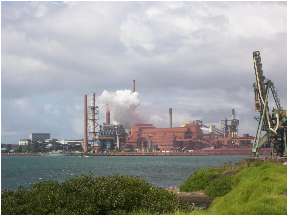
Figure 11 Land uses (BlueScope Steel) looking south of Allotment 5
