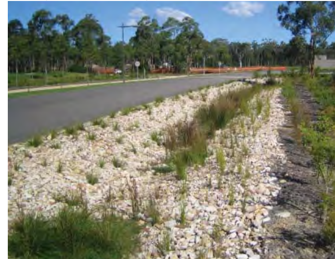
09 (above) & 10 (below) - bioretention swale with sandstone spillings & swale planting
