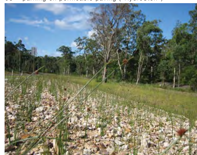
09 (above) & 10 (below) - bioretention swale with sandstone spillings & swale planting
