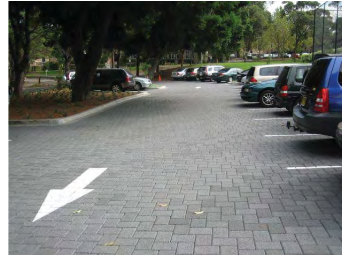
08 - parking on permeable paving ("HydroSton")
