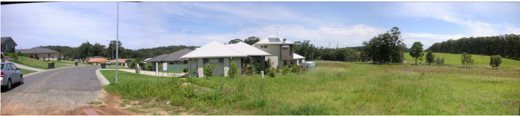
Photo 3: View east to south-east to south Rutland Street
