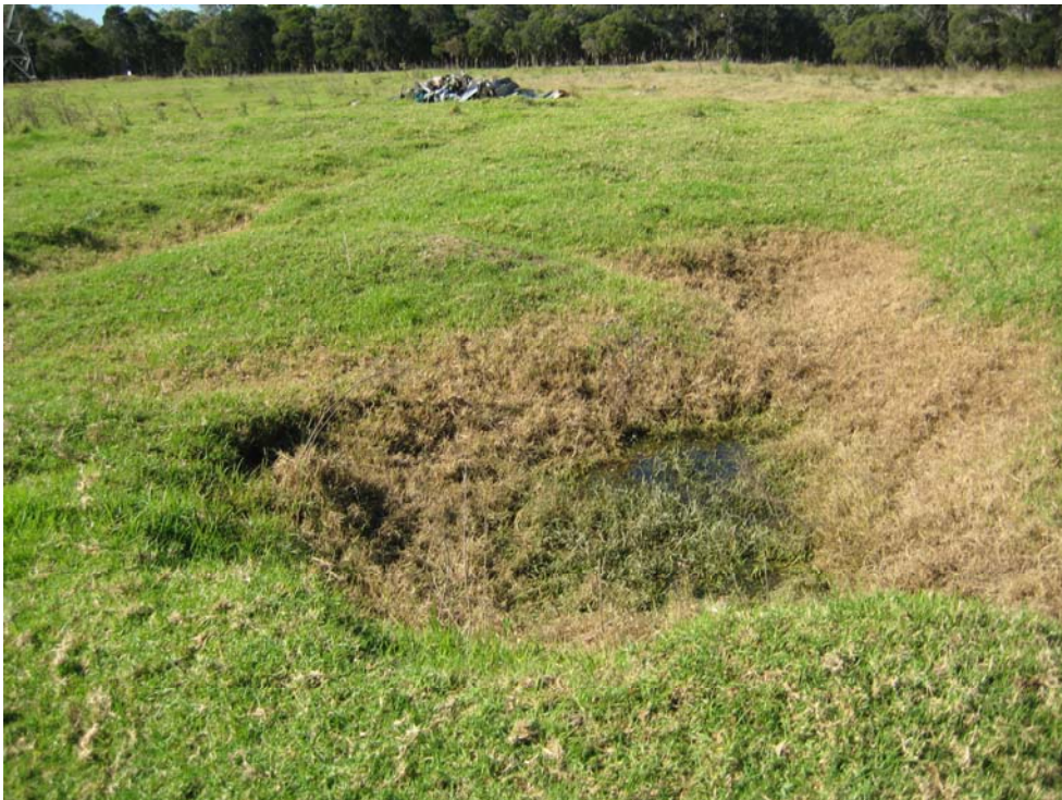
Photo 4: Hummocky ground within southern portion of site looking east (note construction waste stockpile in distance)
