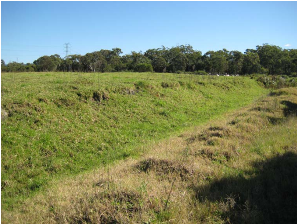
Photo 9: Extent of existing fill ~1m height along north western boundary
