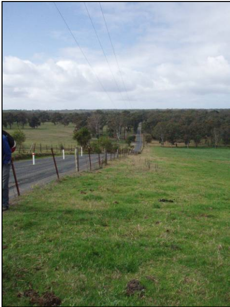
Figure 4.1 View of southern side of existing access road (facing east towards Appin Road).
