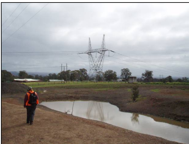
Figure 4.5 View of northern side of existing access road (facing northwest).
