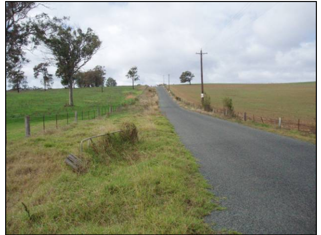
Figure 4.4 View of northern/southern sides of existing access road (facing east).
