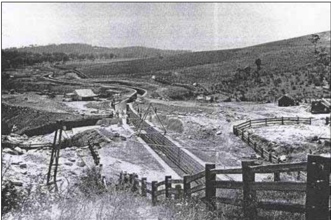
Figure 3.10 View of the Upper Canal under construction c.1886 near Sugar Loaf, note also the primitive huts and humpies erected by workmen as shelter (Higginbotham et al 1992:13).
