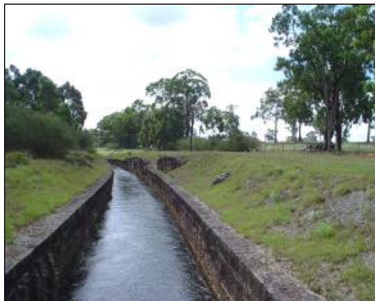
Plate 6.6 A typical portion of type two open canal from section 3 of the Sydney Water Supply Upper Canal, showing square sided masonry walls.
