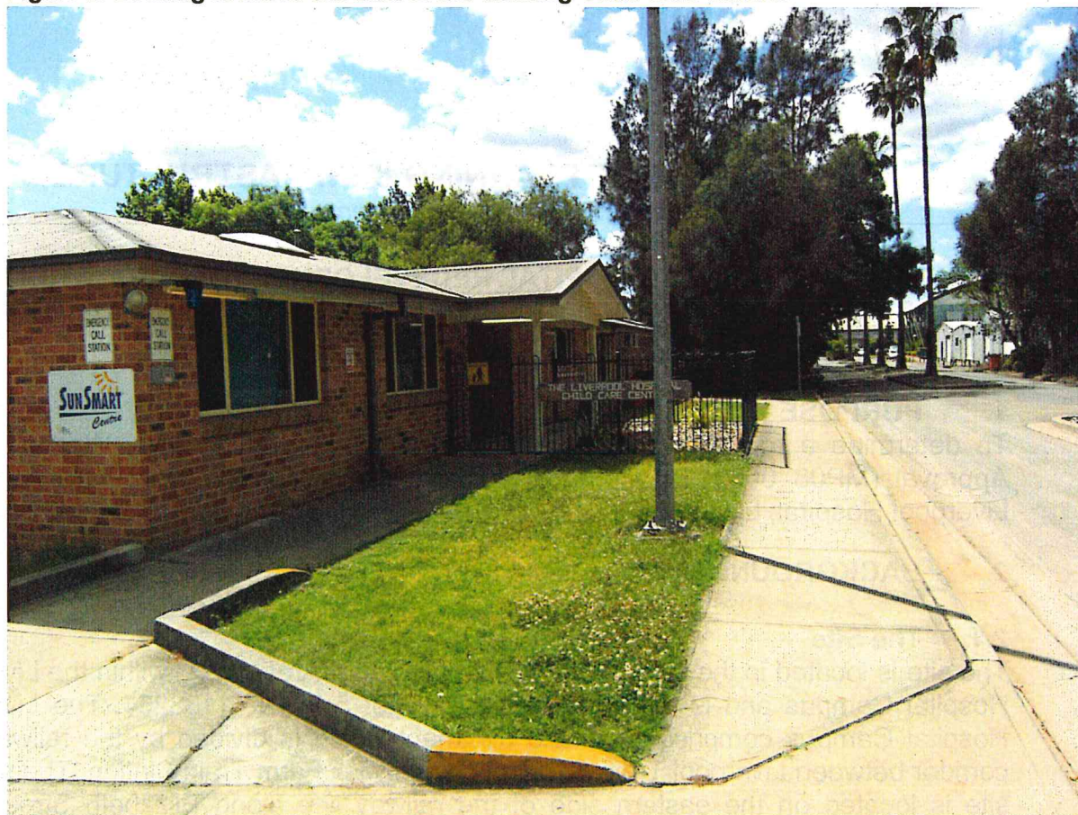
Figure 2: Looking towards the east of the existing Child Care Centre.
