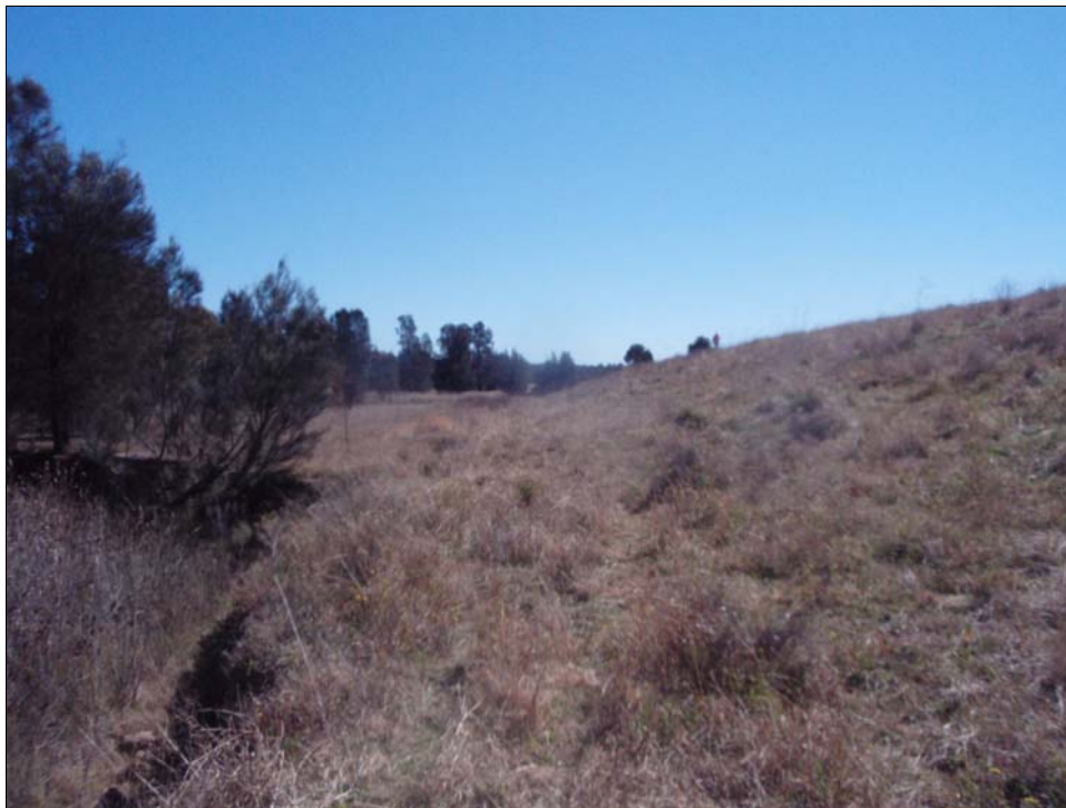
Plate 2 Survey Section 8.5, facing N, route to run on W side of bund wall
