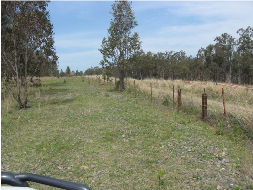
Photograph 13: Ballast surface fill between Ch 228460 and Ch 228580 on Lot 89.
