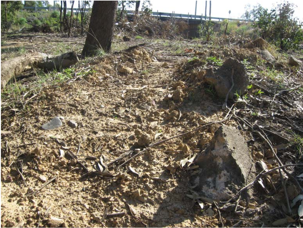
Photograph 19: Fill in north part of Lot 100, note the concrete in the fill.
