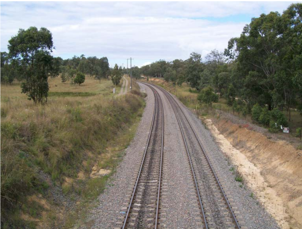
Photograph 2: Location 1 - Looking East from Golden Highway Overpass
