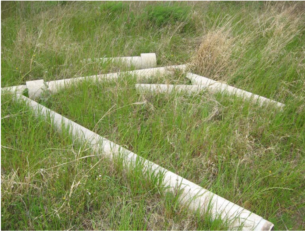
Photograph 7: NW portion of Lot 1 on DP 86239, potential asbestos containing pipes adjacent to acquisition area.
