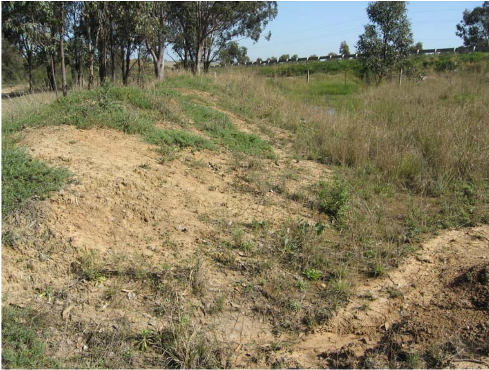
Photograph 21: Drainage swale with earthen embankment in northern portion of Lot 100.
