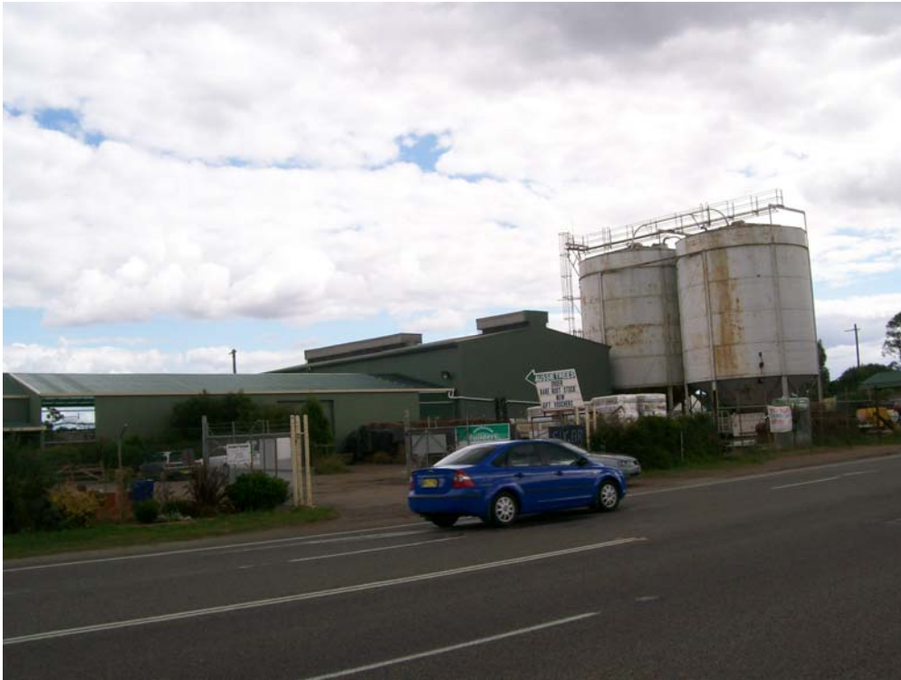
Photograph 3: Location 2 – Aussie Trees looking south from New England Highway
