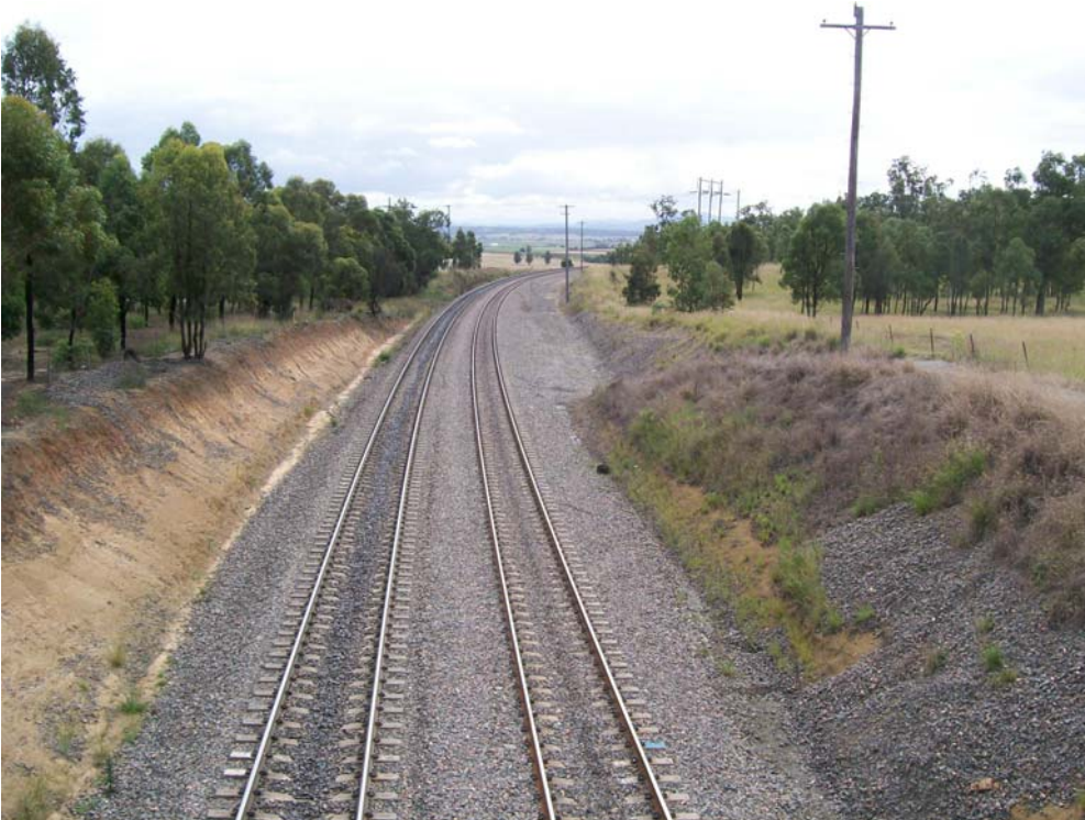
Photograph 1 Location 1 - Looking West from Golden Highway Overpass
