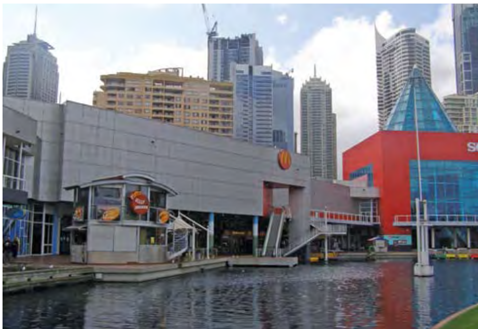
Figure 5 – View of mid section of existing building
