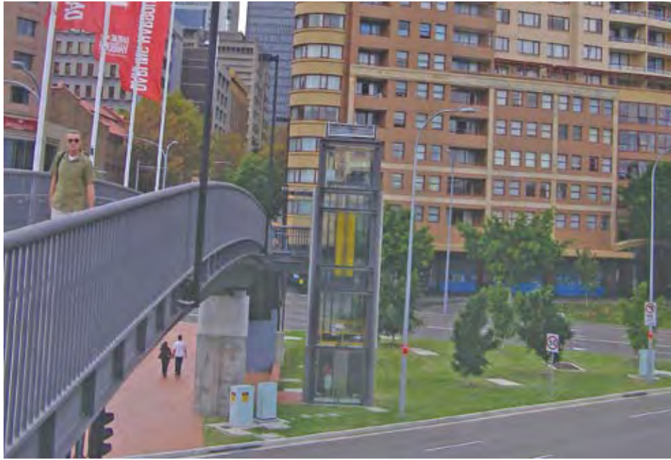
Figure 8 – Bathurst Street pedestrian bridge and lift over Harbour Street
