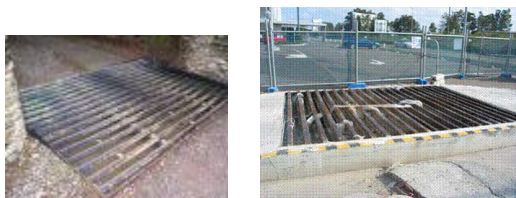
Figure 5.1 Possible solutions to sediment lost via motor vehicles.
