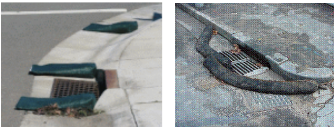
Figure 5.3 Common commercial systems preventing sediments entering drains.
